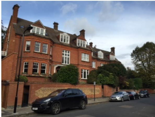
3 Nutley Terrace. Note the symmetrical arrangement of the bay windows.
