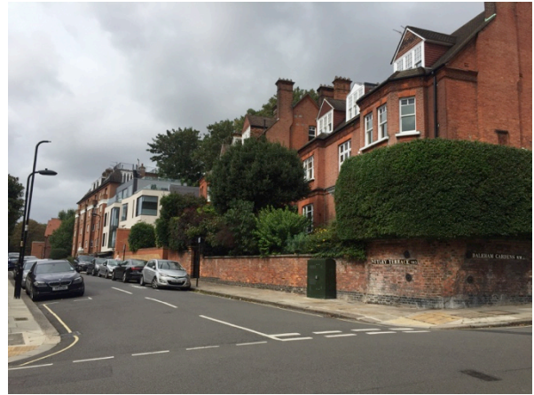
Historic villa on north side of Nutley Terrace at corner of Daleham Gardens. Note the symmetrical bay window arrangement.
