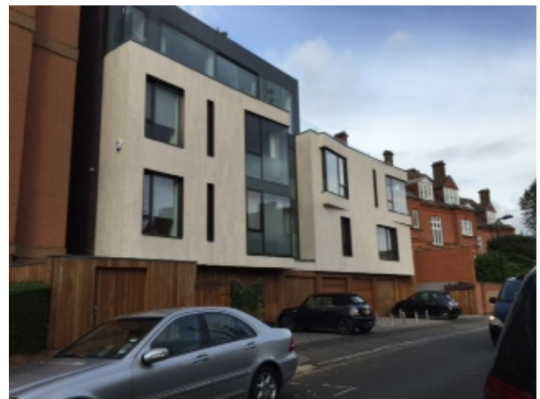
5 Nutley Terrace, modern development that does not reflect the materials, roof forms or sizes and proportions of the historic buildings.
