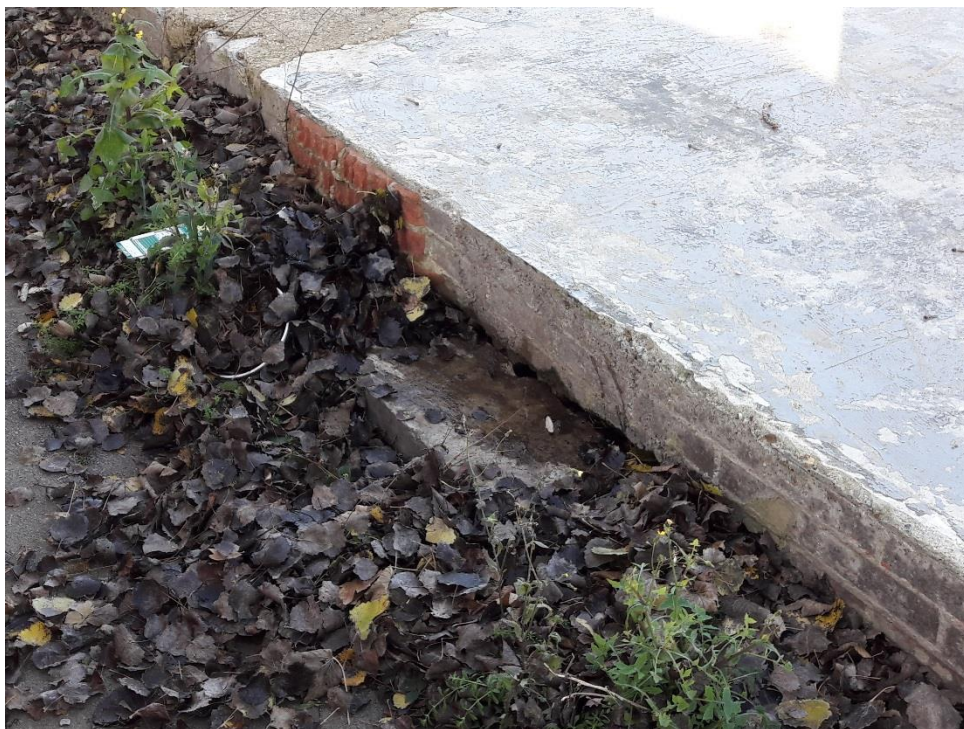
Photo 2: Showing edge of slab to be removed.
