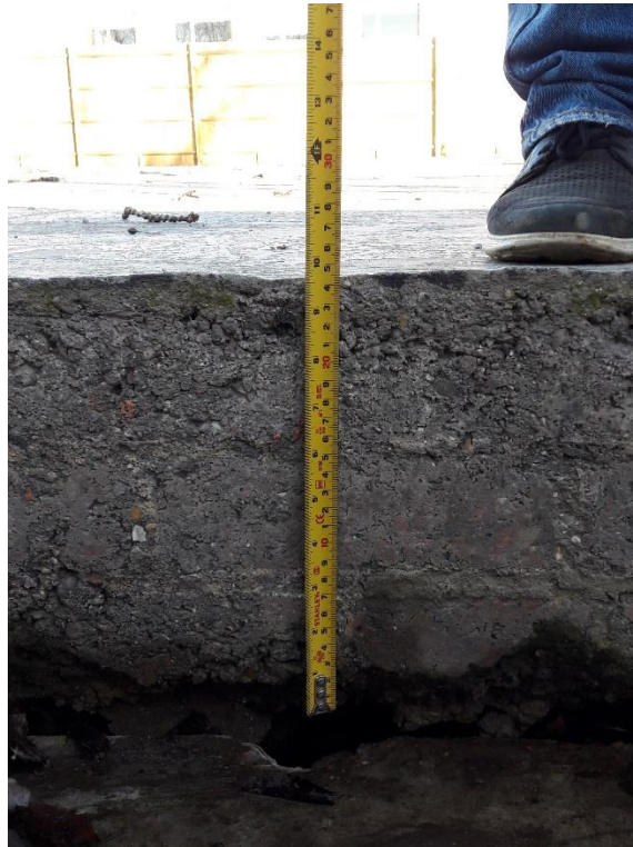
Photo 3: Edge of Slab to be removed depth 250mm
