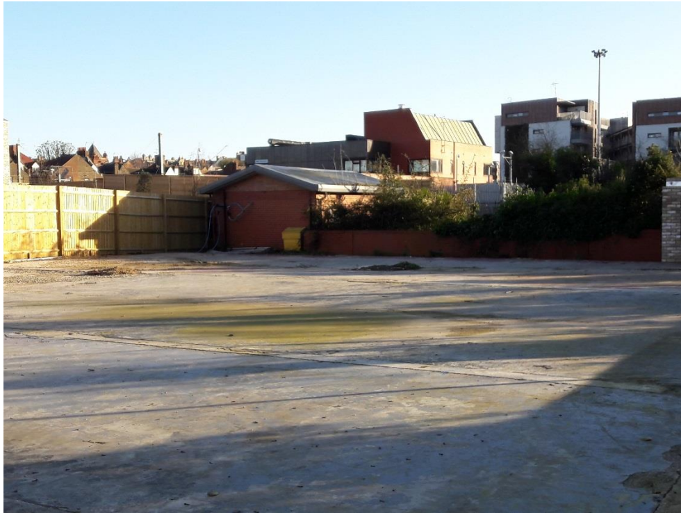
Photo 1: Showing current site and extent of existing concrete slab.
