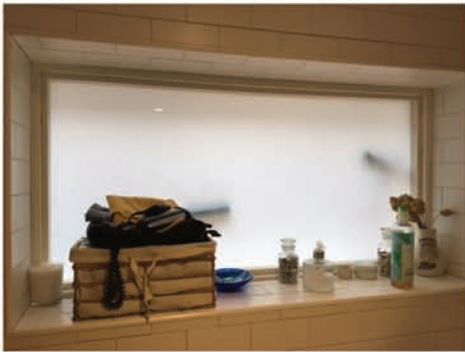
Fig. 20 - Internal window in basement shower room
