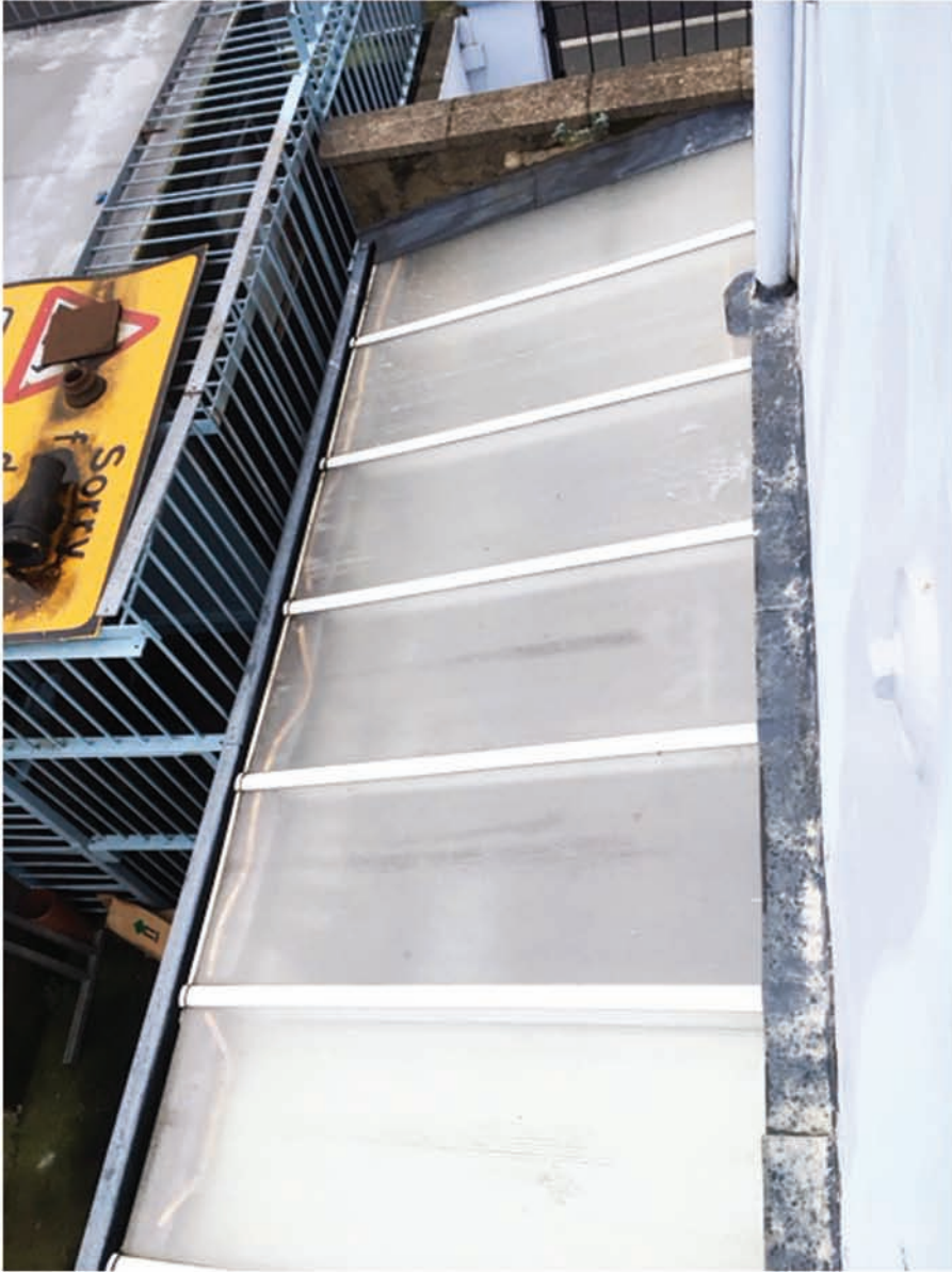
Fig. 15 - View of existing Polycarbonate Roofing to side addition
