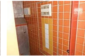
ACCESS PANEL TO MH 3.JPG
