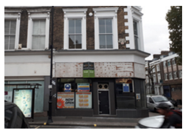
VIEW FROM KENTISH TOWN ROAD
