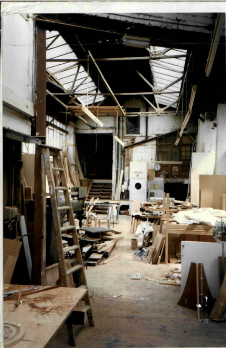
INSIDE REAR SHED
