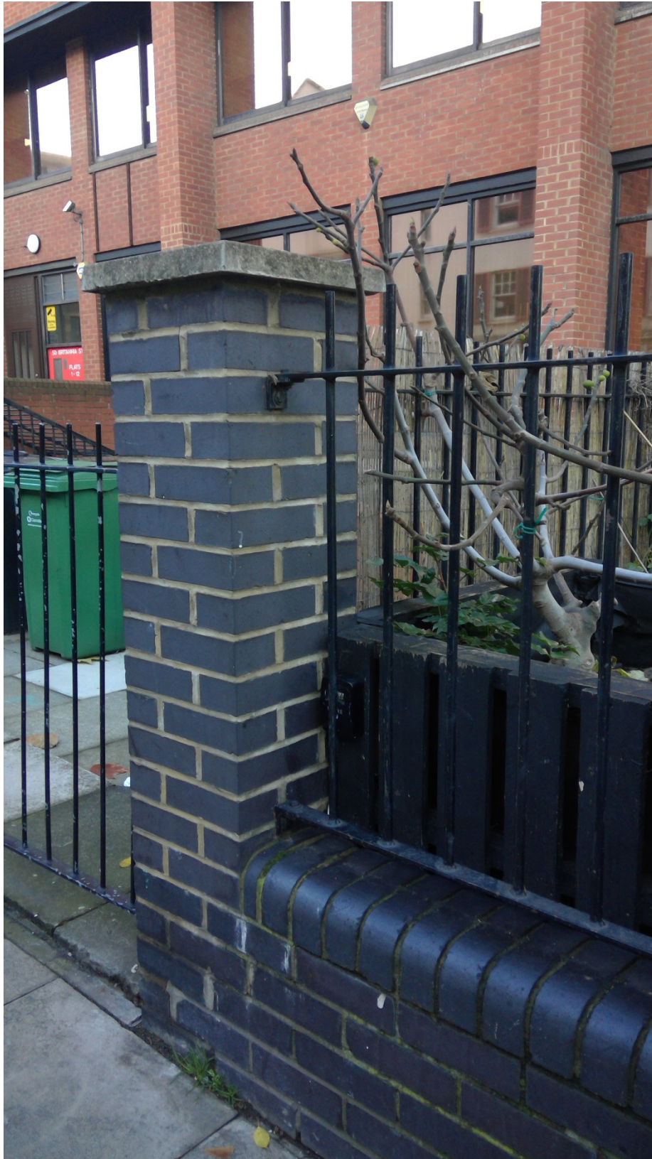
Detail of existing railing and pier
