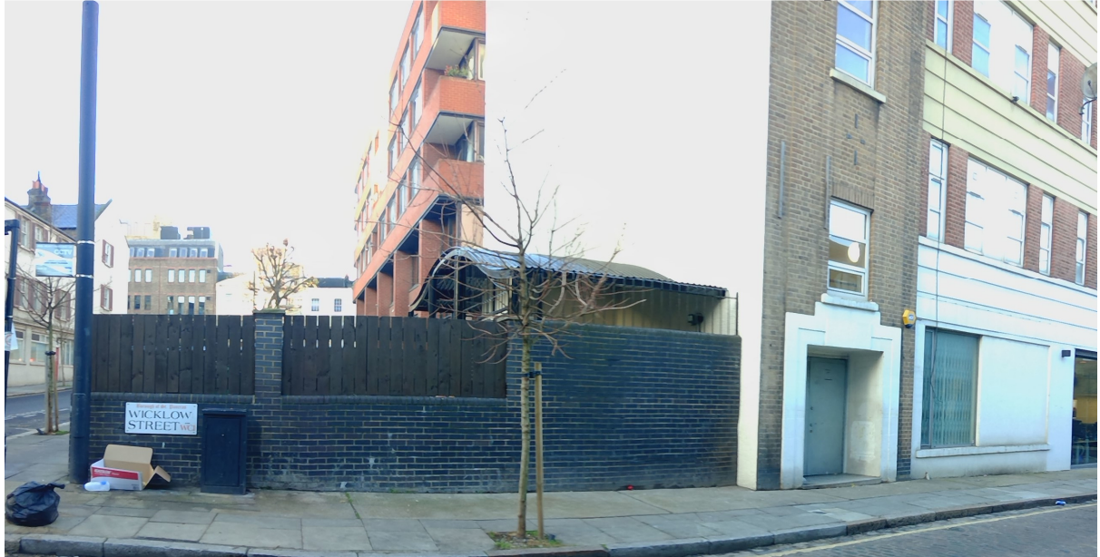
Right side elevation – Timber fence panels are to be replaced with metal railings as per the front elevation.
