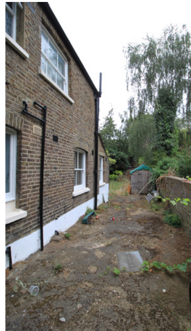
View to rear garden from side passage
