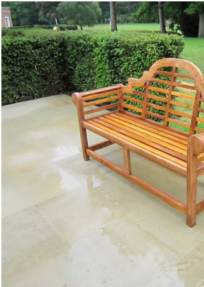
York stone paving to match existing
