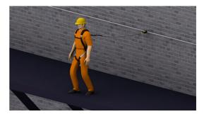
If fitting a fall restraint system, it is recommended that the system should be tested to fall arrest loads to ensure a person's safety in situations where the system may be misused (i.e. when the person using it wears an over-length lanyard to enable access to the edge of a roof).
