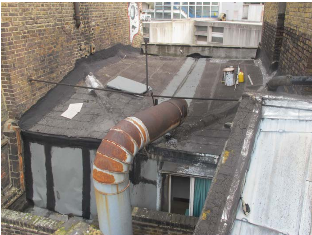
View of the rear of the site- butterfly and mansard roof, 2014
