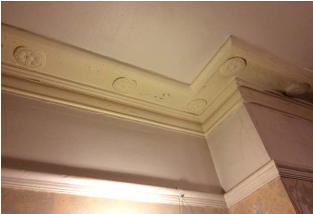
Example of a flat-run bed cornice, c. 1830s, Lofting Road, Islington
