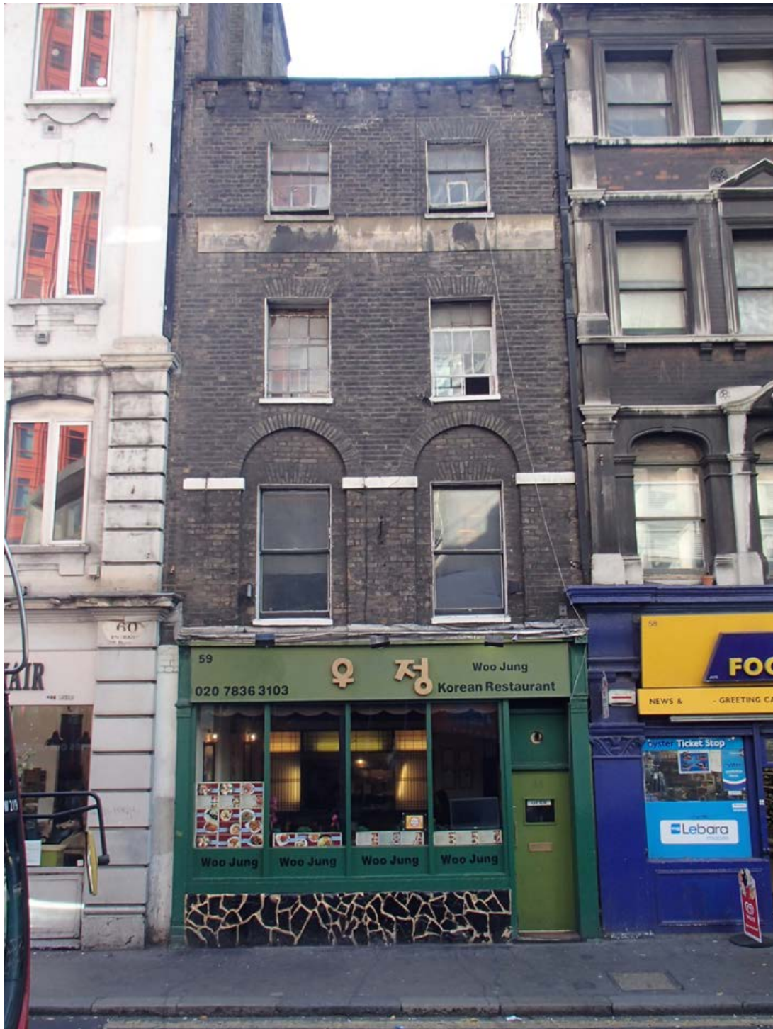
Street elevation of No. 59 St Giles High Street in 2014
