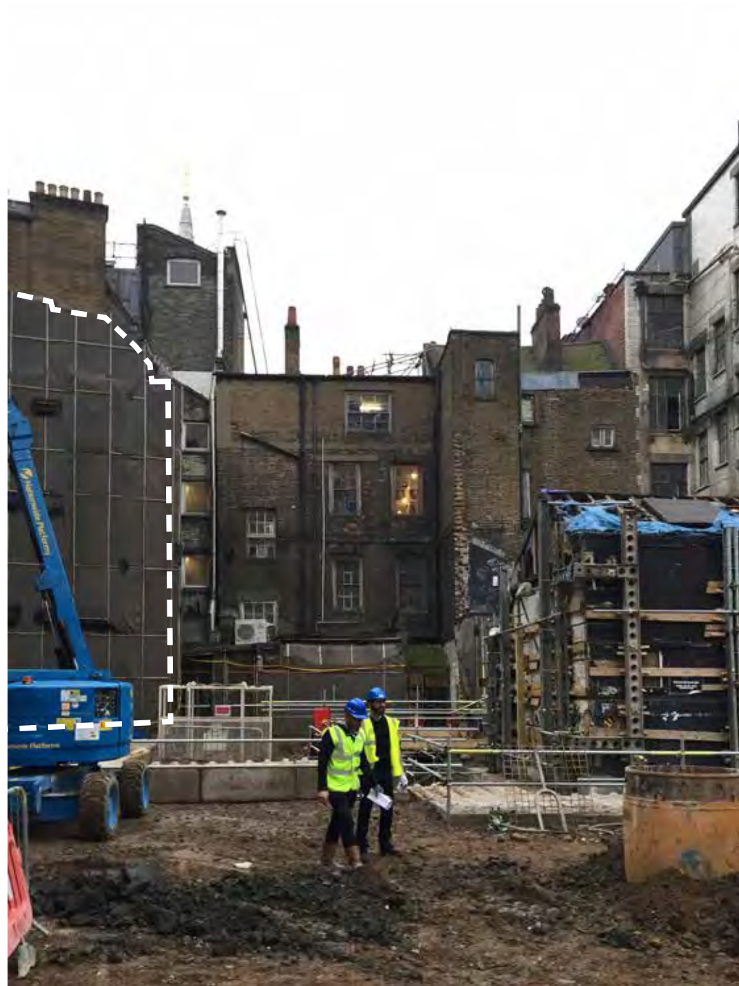
Image showing the exposed party wall of 59 St Giles High Street, with strengthening straps, weather protection and battening visible
