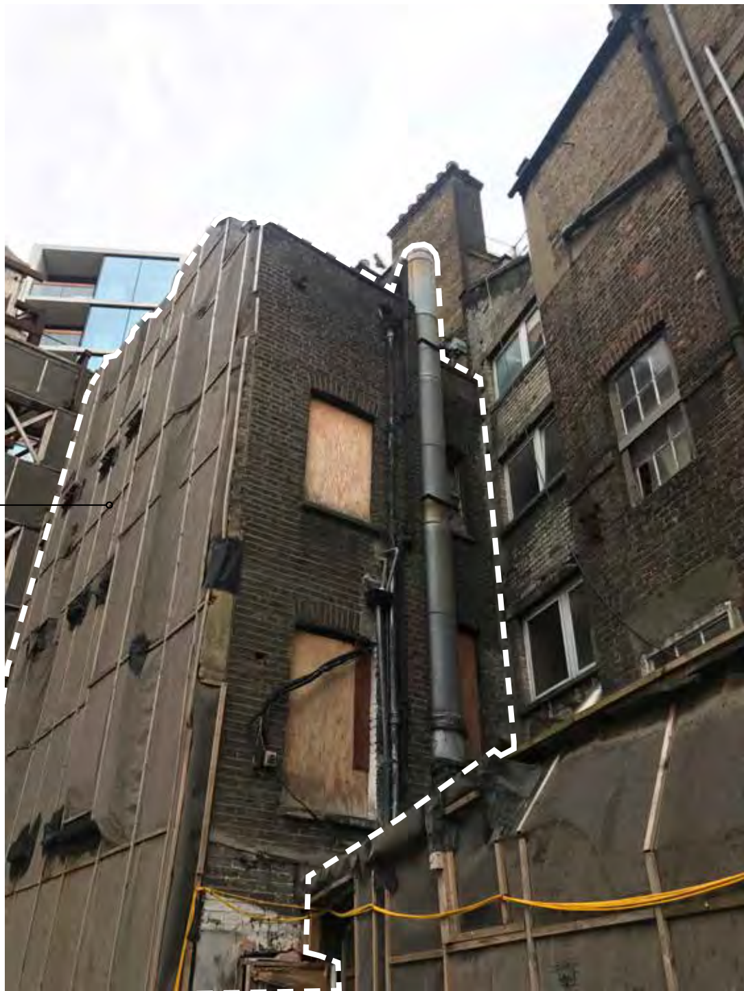
Image showing the rear elevation of 59 St Giles High Street, with windows boarded up. Large extract duct from ground floor to roof visible.
