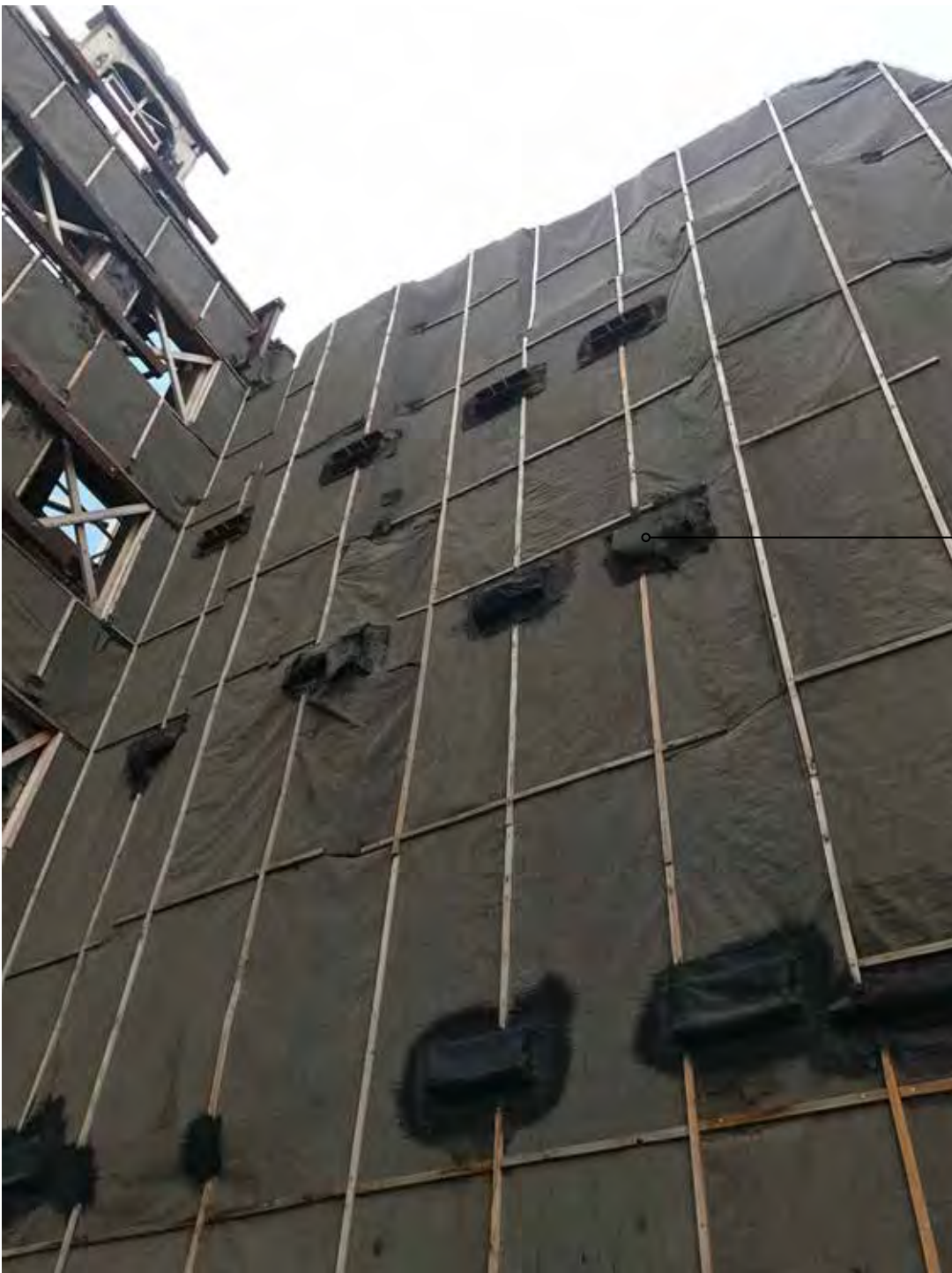
Image showing the exposed party wall of 59 St Giles High Street, with strengthening strapping visible
