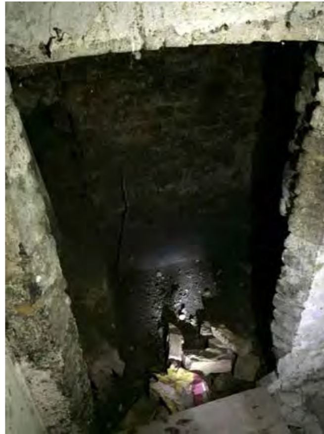
7 - Original coal store in in-filled yard to the rear
