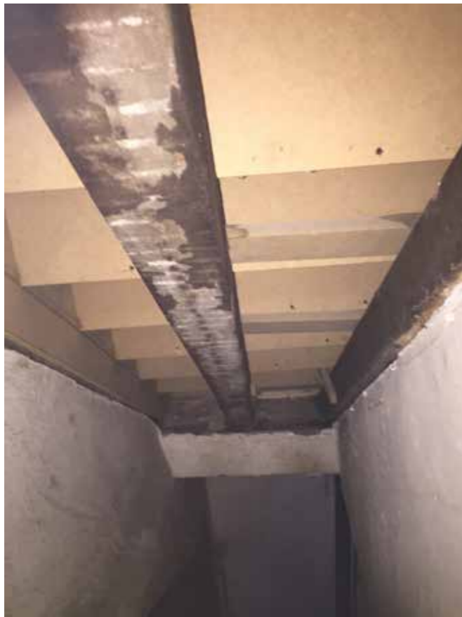
12 - Underside of MDF stair from ground to first floor
