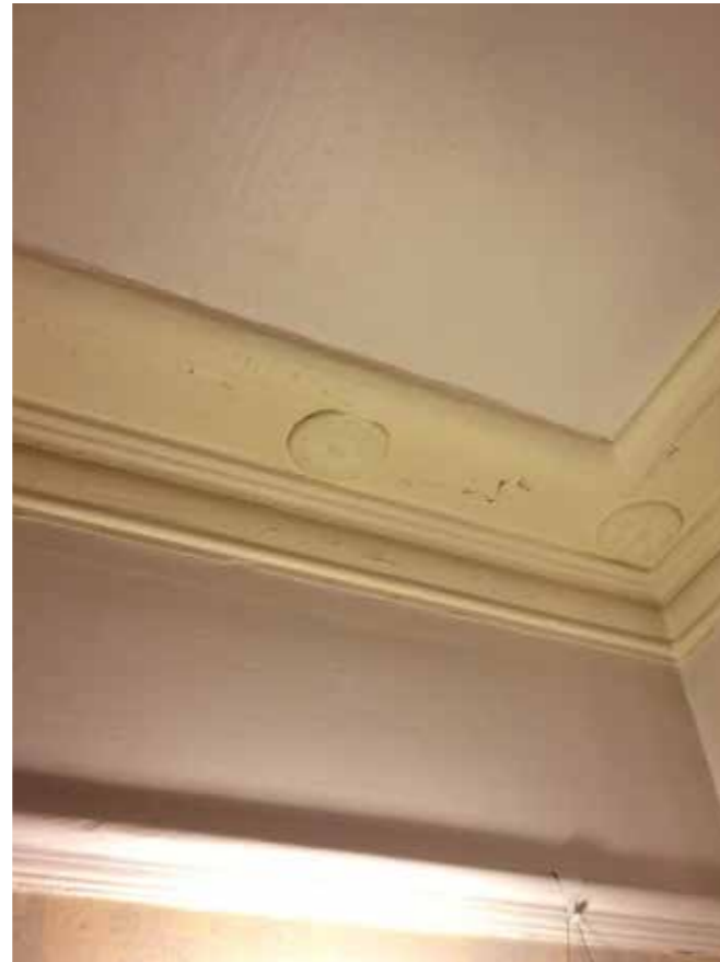
26.5 - Precedent Cornice, House in Lofting Road, c1840
