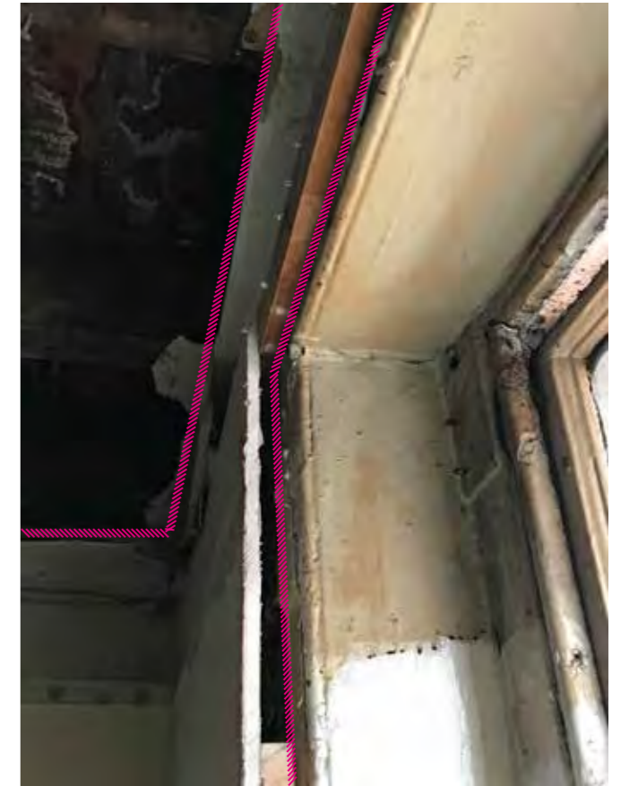
30 - Detail of layered faces of internal wall
