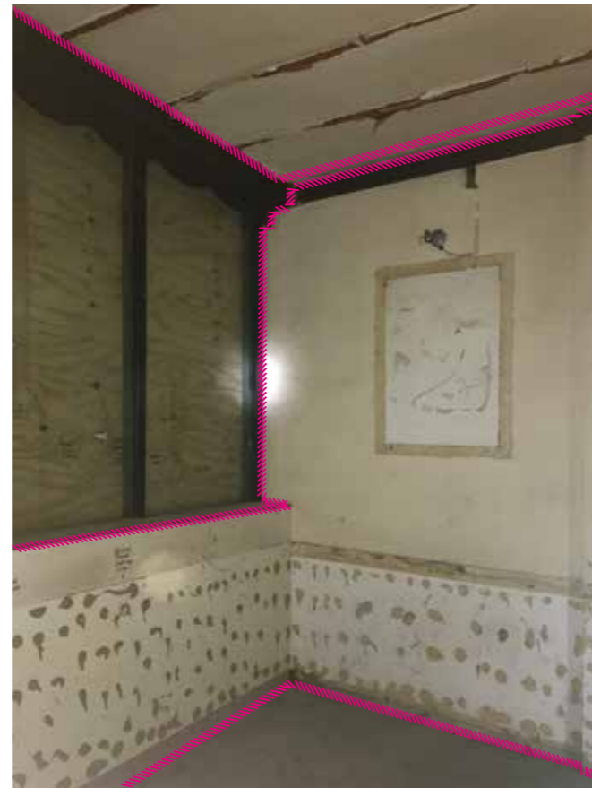
13 - Shop front boarded up
