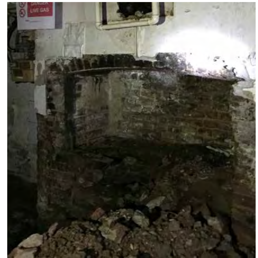
5 - Chimney stack and opening in primary room.
