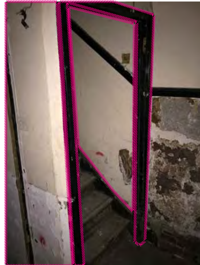
25 - Stair up to floor above.
