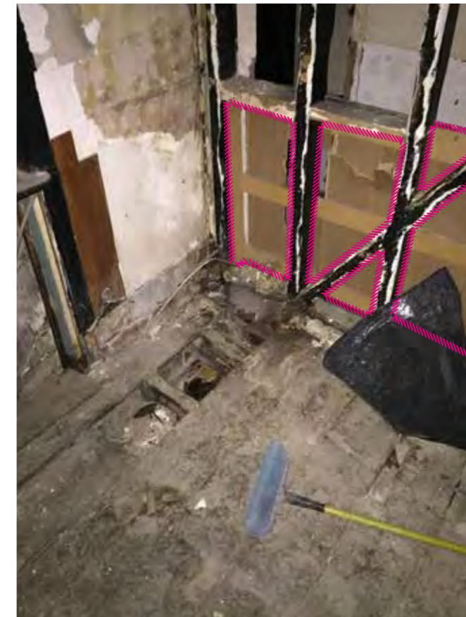
22 - Floor joists in rear room
