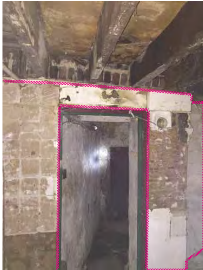
6 - Original back door to yard - now infilled through to coal stores.
