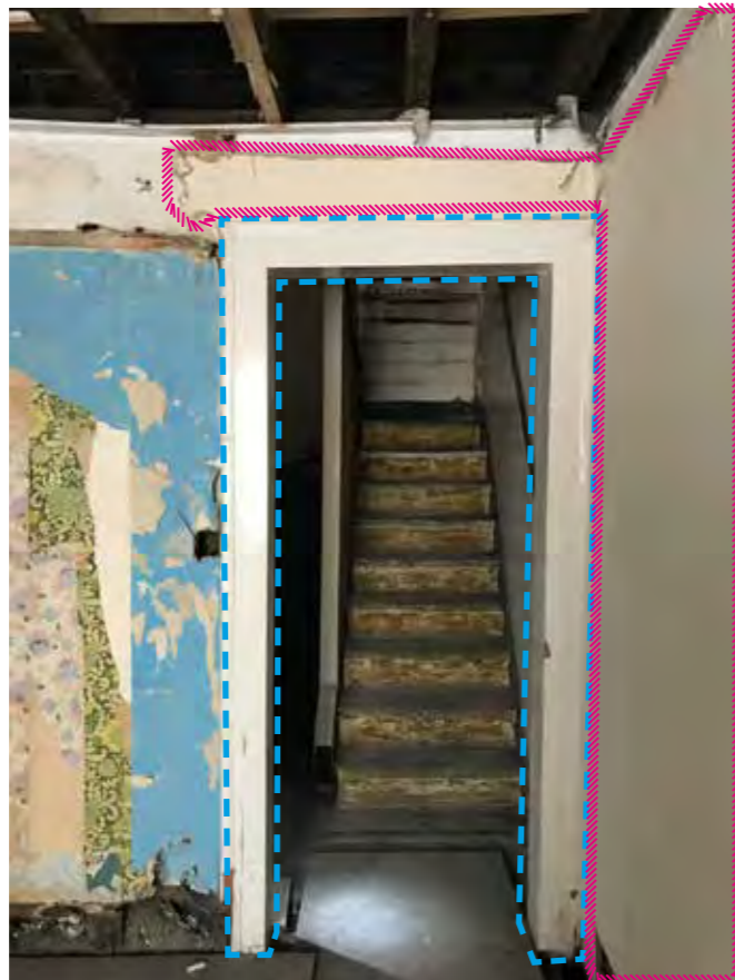
34 - Original opening and architrave between primary room and stair. Unoriginal osb / chipboard staircase visible. Multiple layers of patterned wallpaper
