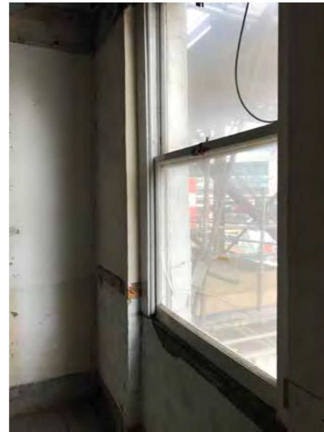
18 - Detail of window opening. Unoriginal single pane sash window, inappropriate to building period.
