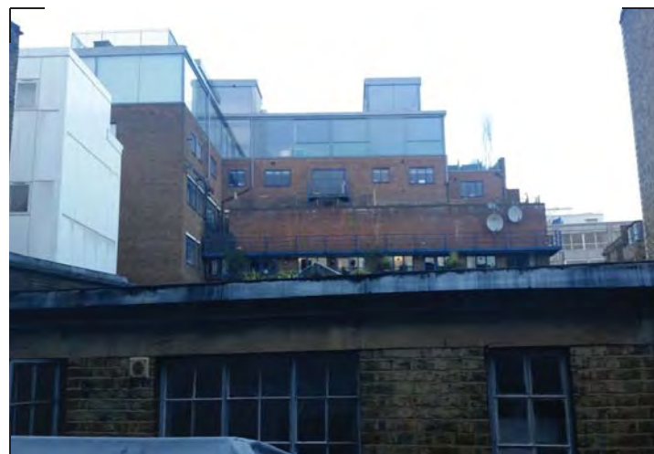
View from roof at rear of site looking North
