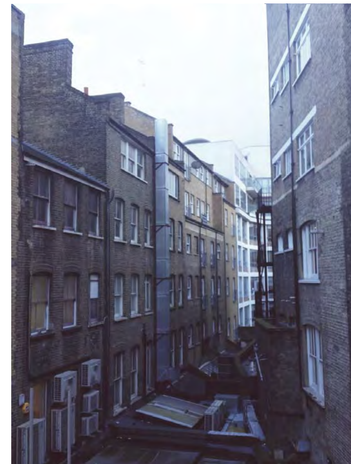
View from roof at rear of the site looking South
