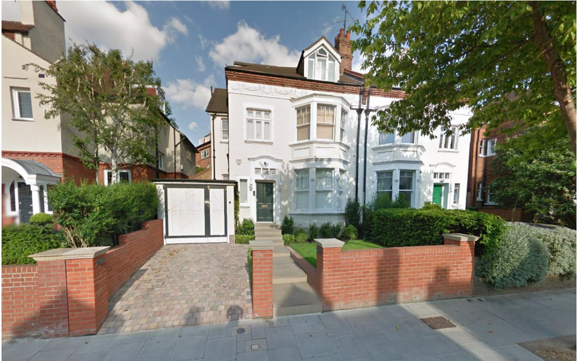
Figure 13. New brick wall with piers and coping stone finish at 30 Hollycroft Avenue.
