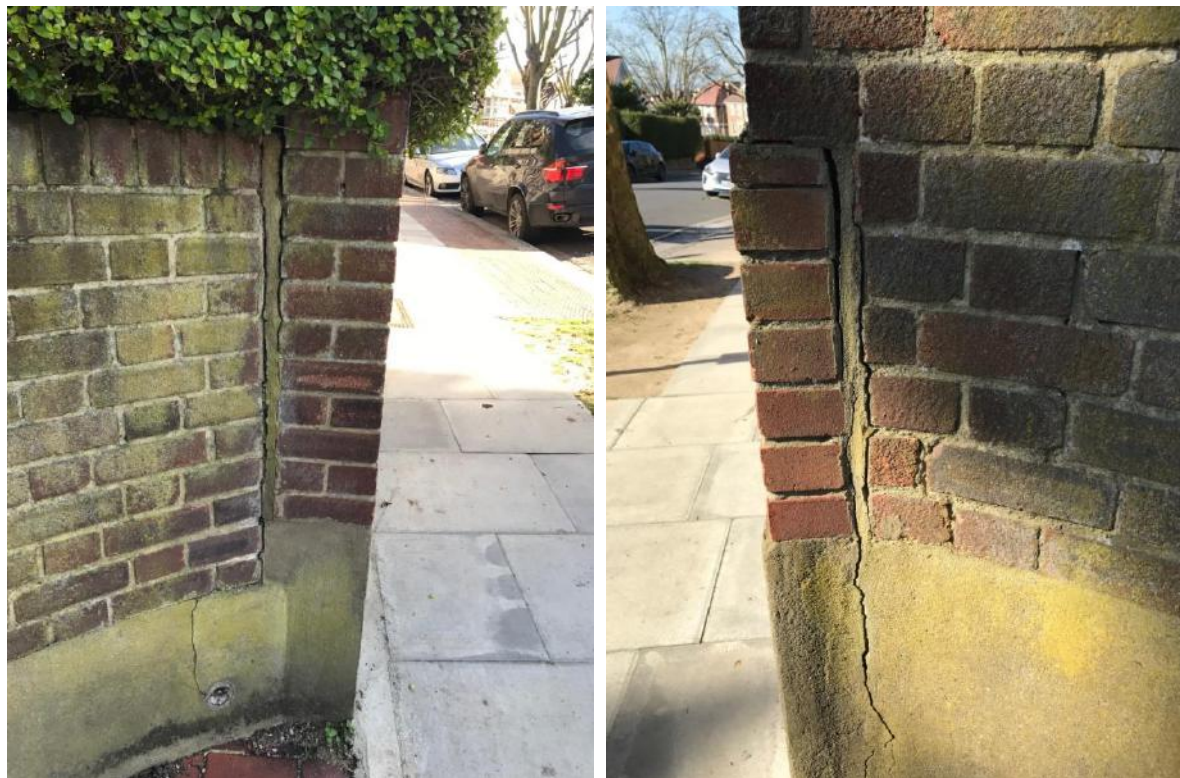
Figure 11. Damage to the existing front boundary wall.
