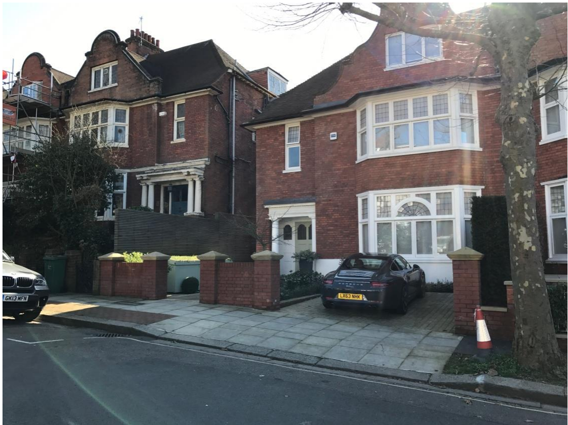
Figure 13. New brick wall with piers and coping stone finish at 30 Hollycroft Avenue.
