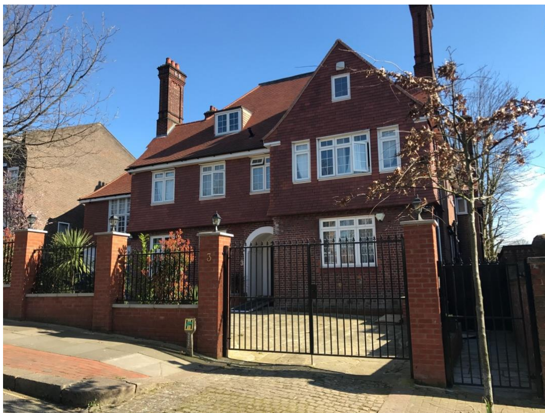
Figure 15. Brick front boundary wall with black metal railings and piers with a coping stone finish at 3 Oakhill Avenue.
