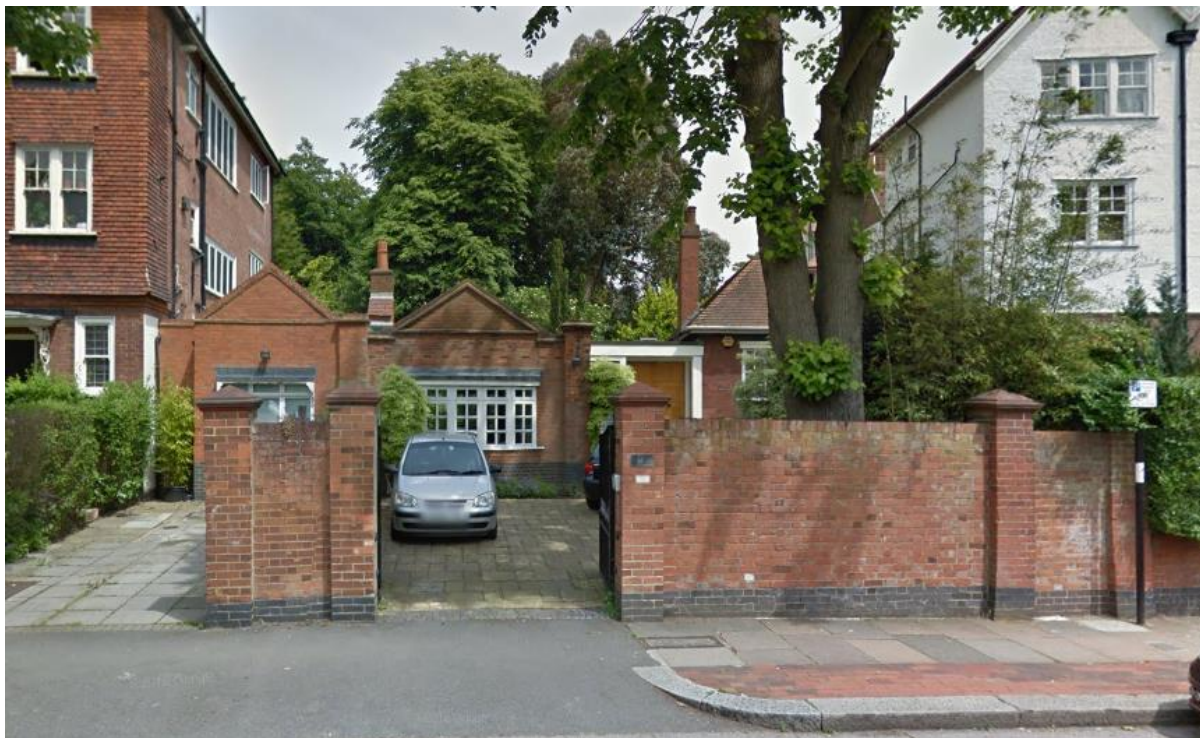
Figure 15. Brick front boundary wall with black metal railings and piers with a coping stone finish at 3 Oakhill Avenue.
