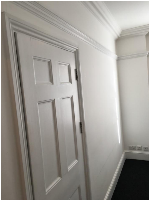
Wall between Room B and Room C as seen from within Room C. This wall would have a large opening made in it, but would retain a downstand with picture rail. Nibs either side of the wall would also be retained.
