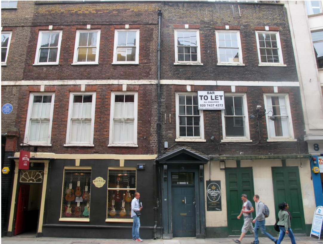
Figure 1: Nos. 6 and 7 Denmark Street
