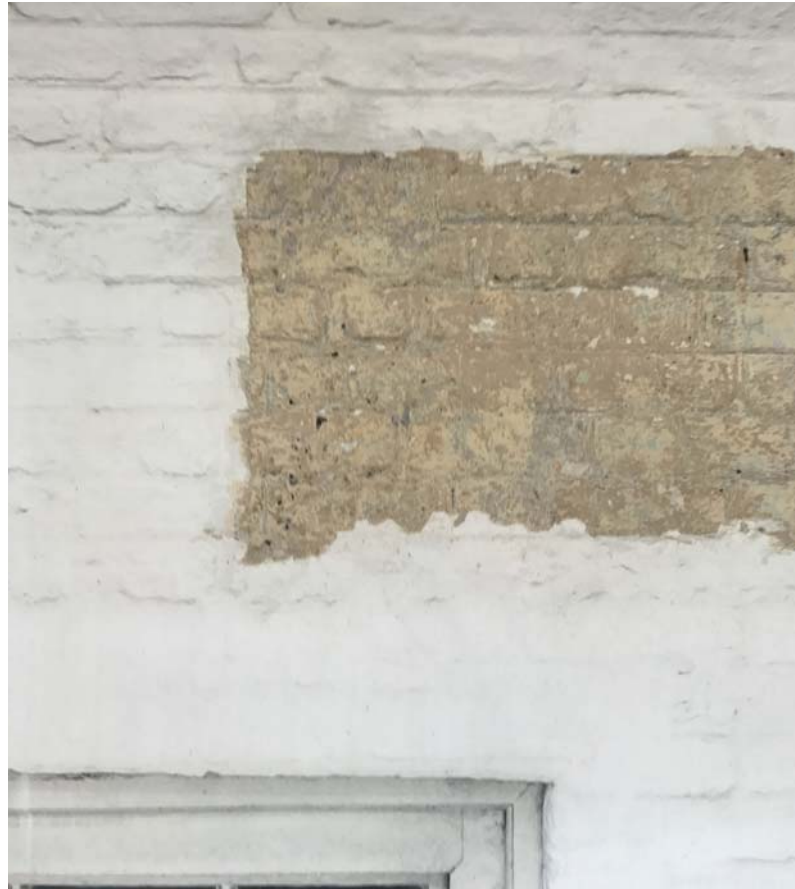
No. 10 Denmark Street, paint removal test area using Peelaway, September 2017
