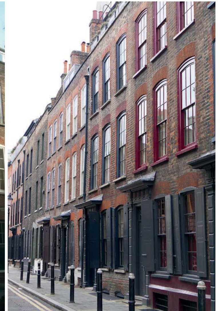
Terrace of townhouses on Wilkes Street, Spitalfields, built 1721-22
