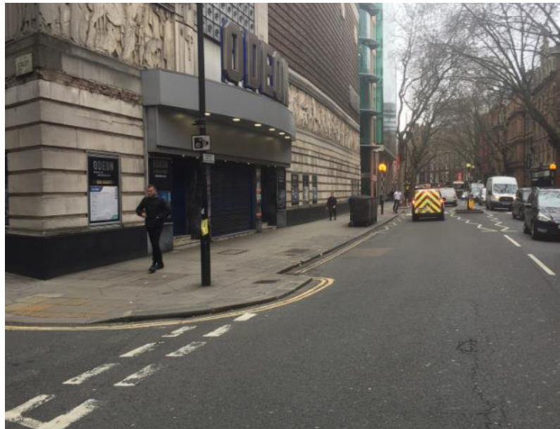
Figure 4: Existing Build Out at Stacey Street / Shaftesbury Avenue Priority Junction
