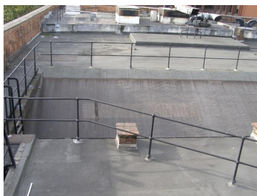
Lined roof space
