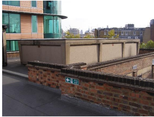
Stores on roof space
