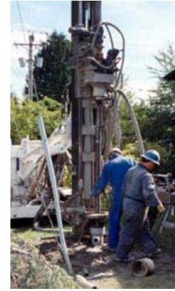
Vertical Pipe Drilling Rig
