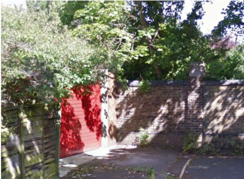
Photograph 2: Brick wall separating T1 from application site (Source: Google Maps)
