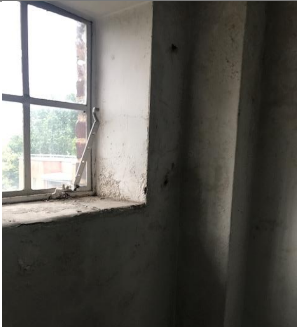
Walls to staircase A
