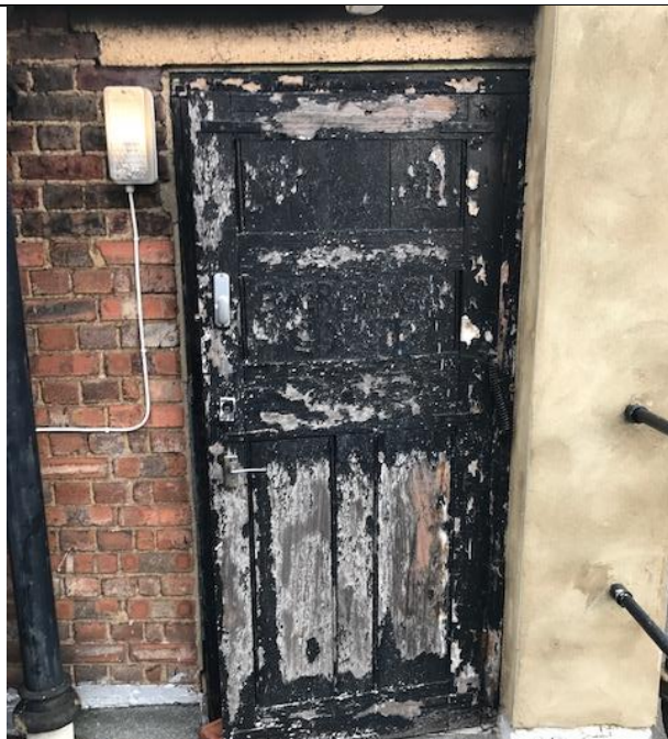
Door leading from staircase A onto roof
