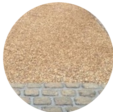
4 Tar and chip surfacing
