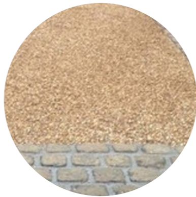
4 Tar and chip surfacing
