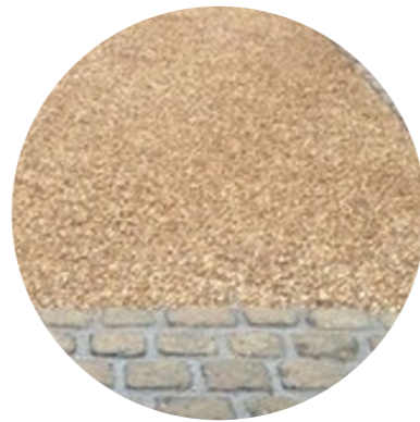
4 Tar and chip surfacing
