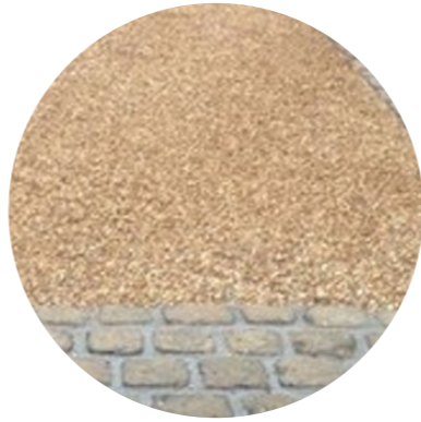
4 Tar and chip surfacing
