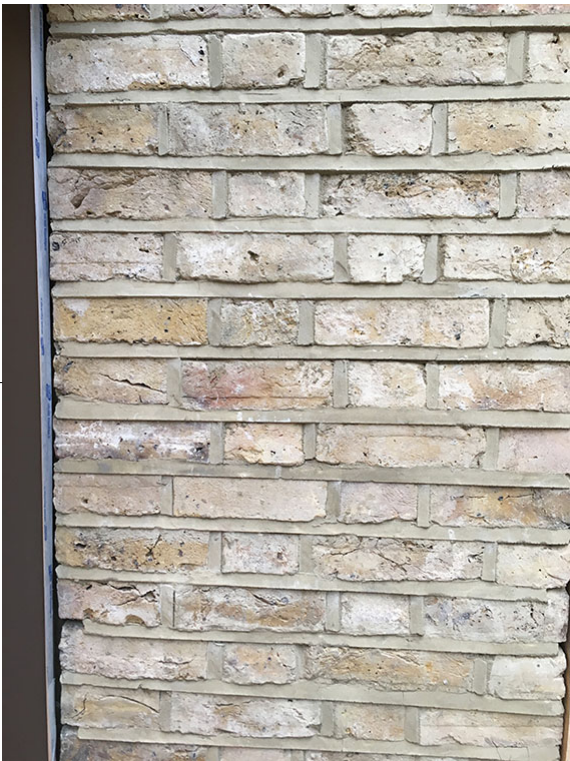
Reclaimed London Stock bricks with weatherstruck pointing to match existing
