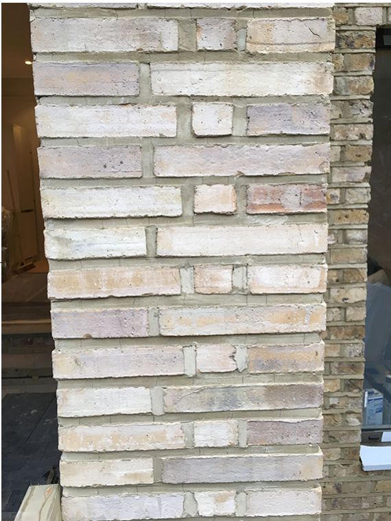
Petersen D72 FF facing brick with recessed pointing to match sample
