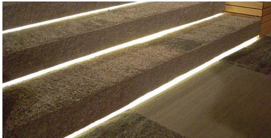
Recessed lighting within step units to back garden
