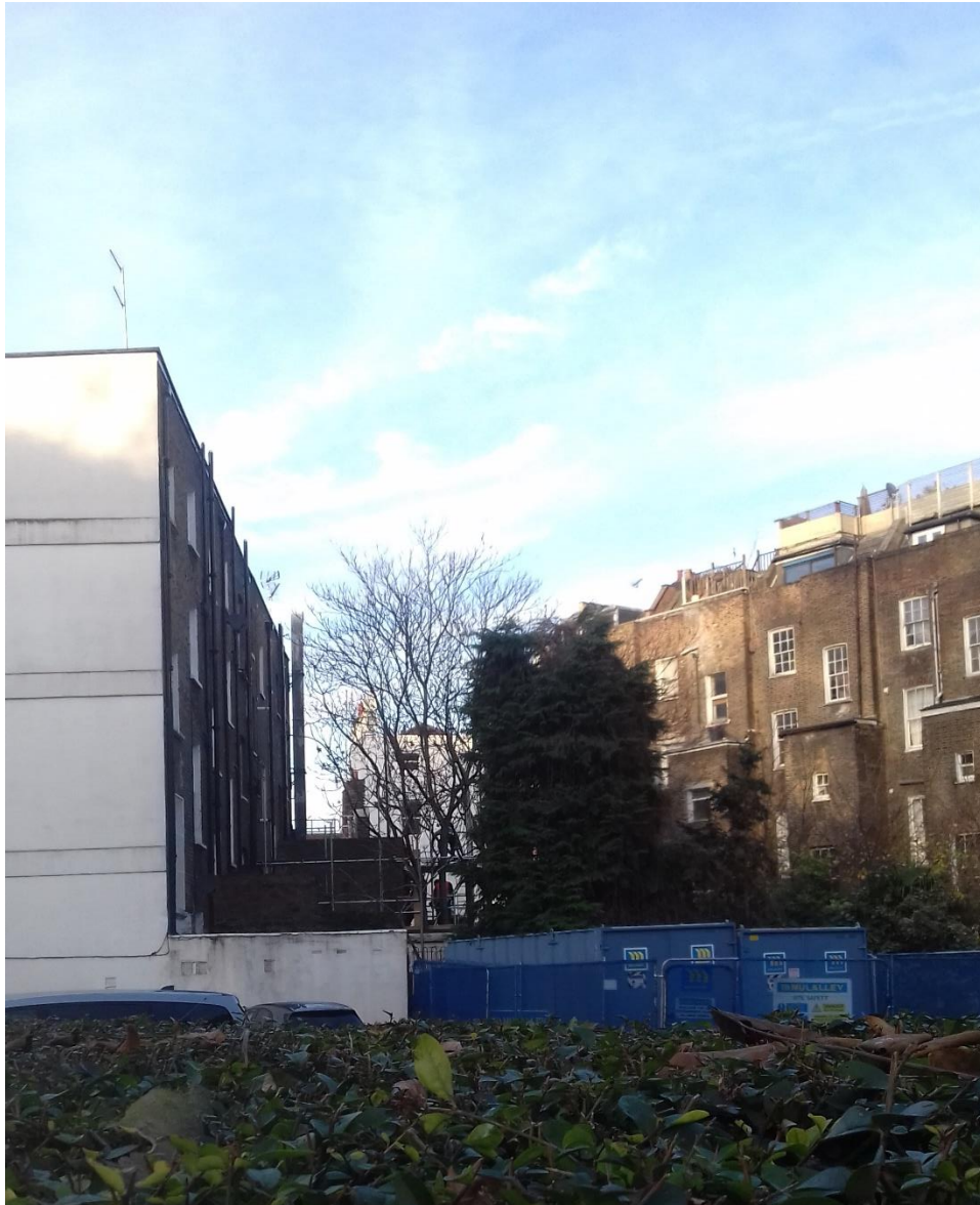
PLATE 3: LOOKING TOWARDS THE REAR OF 1 HURDWICK PLACE
