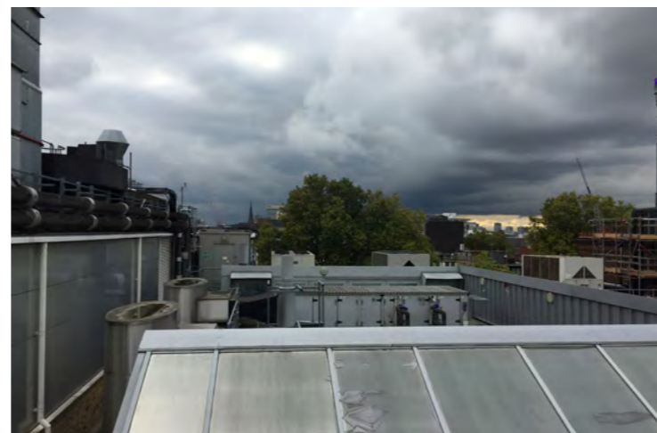
North Courtyard Building Existing Rooftop View
