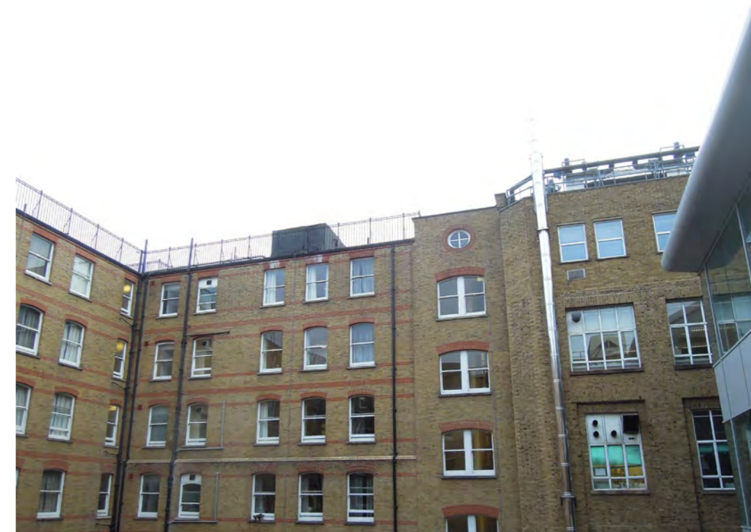
Adjacent Warwickshire House View Facing East
