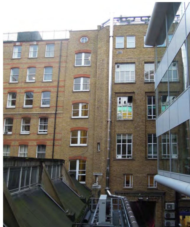
Service Yard View Facing East
