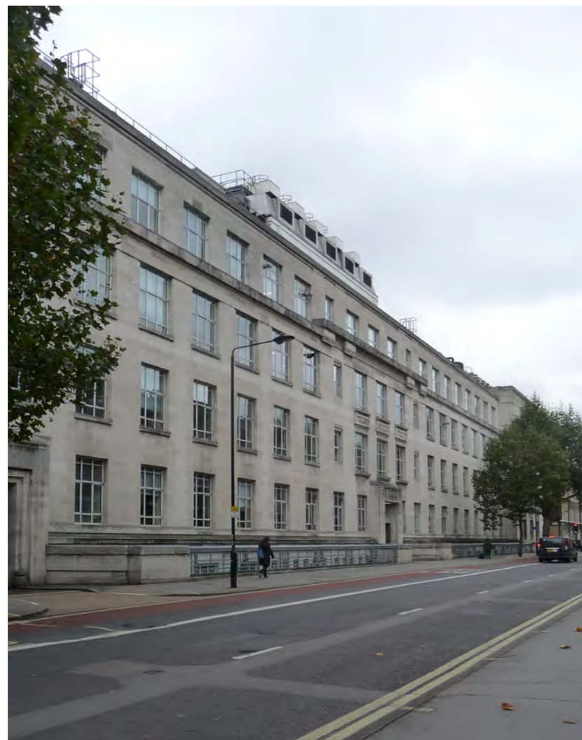
View Along Gower Street Facing South
