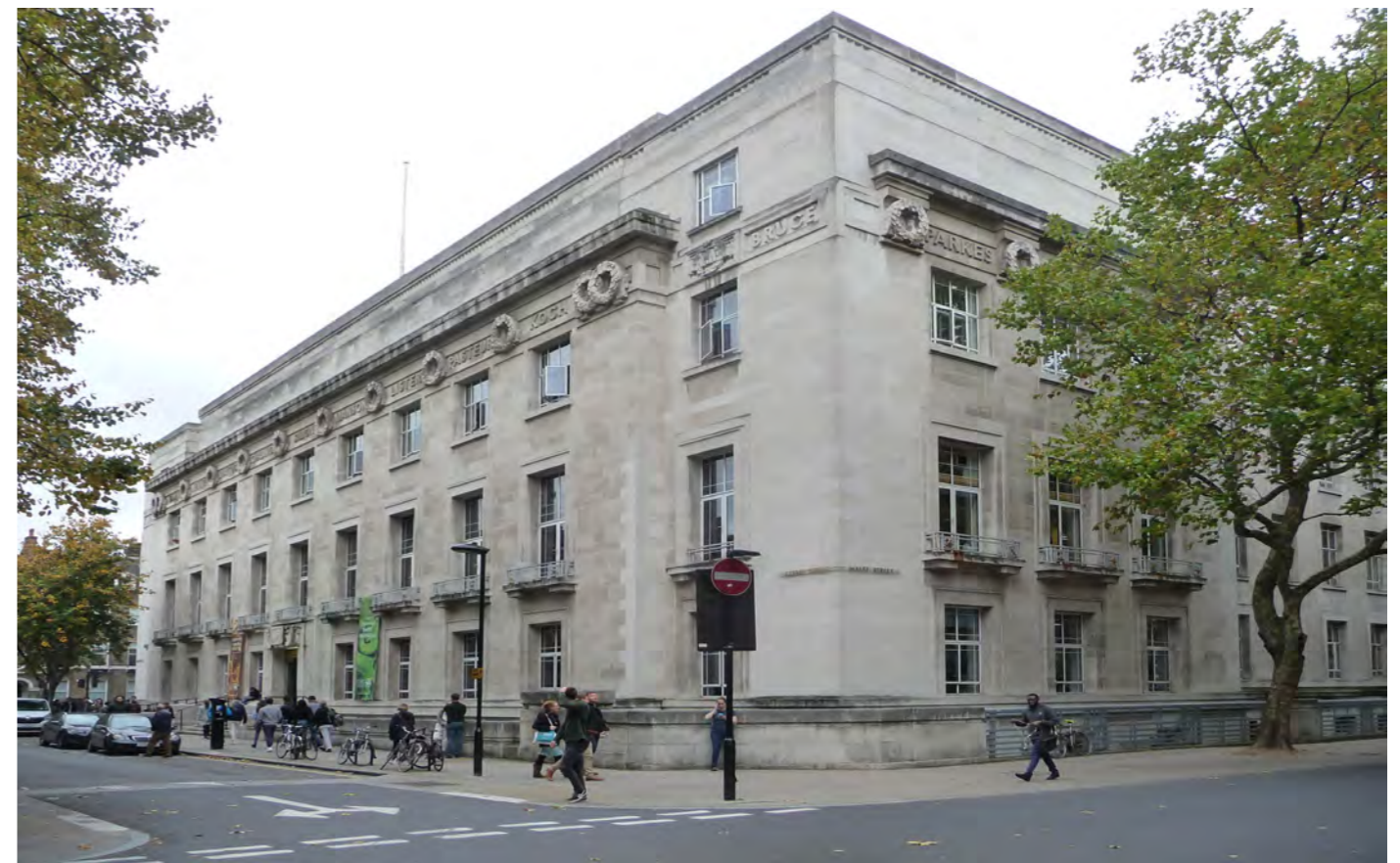
View To Keppel Street Main Entrance Facing East
