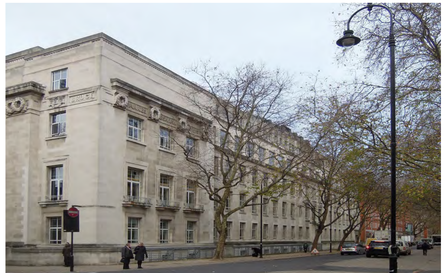
View Along Malet Street Facing North
