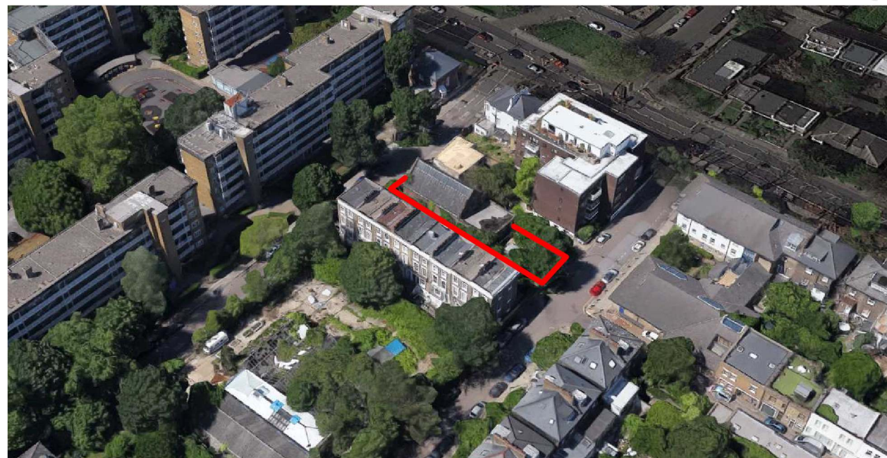
Aerial View Looking East Towards Proposed Development Site
