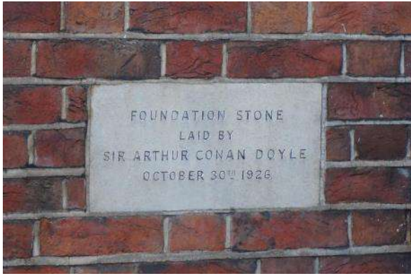
The foundation stone laid by Sir Arthur Conan Doyle
