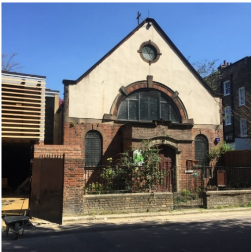
Pic 5 – Existing Building from the South
