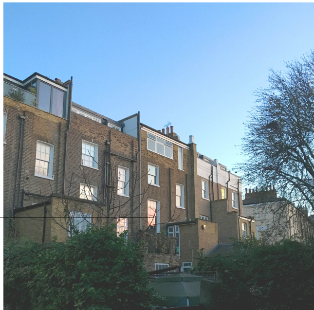
View of rear of 13 Princess Road
