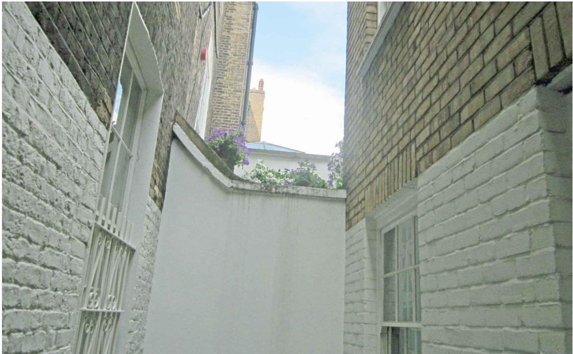
EXISTING BOUNDARY WALL
