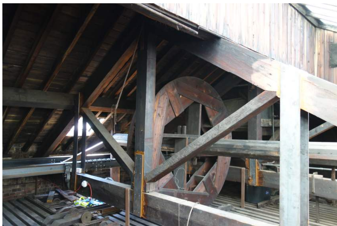
Image 23: View within flytower showing scenographic equipment
