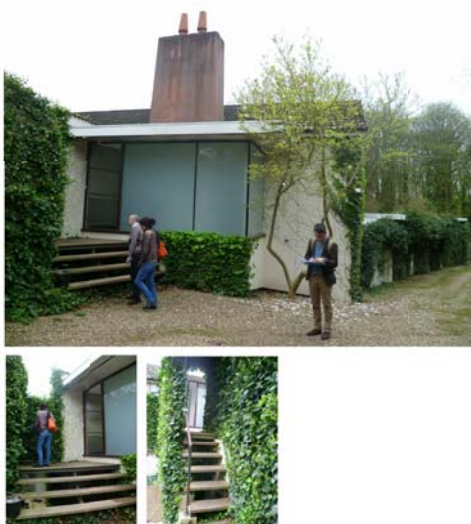
Timber platform/steps (light weight structure) constructed above ground surface level.
