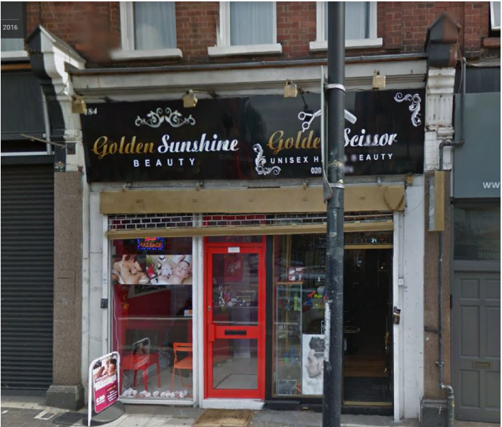
05 Existing Photo NTS
