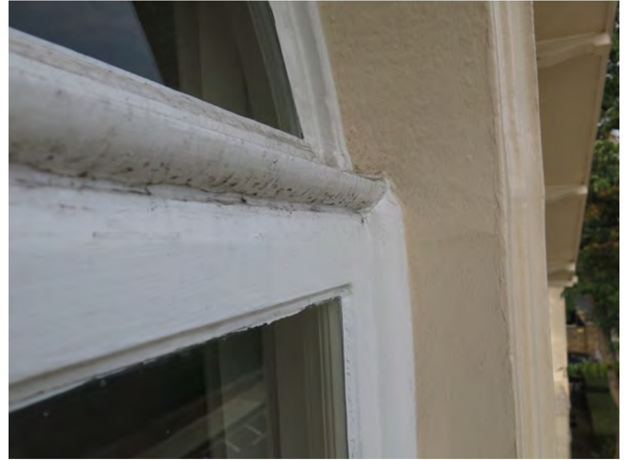
Figure 29: Detail external transom which acts as a cill to shed water from the thicker casement section below. Externally the window is surrounded by a stucco window architrave
