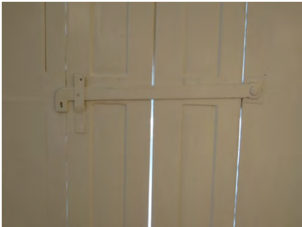
Figure 16: An original shutter stay-bar but the catch is a relatively modern replacement
