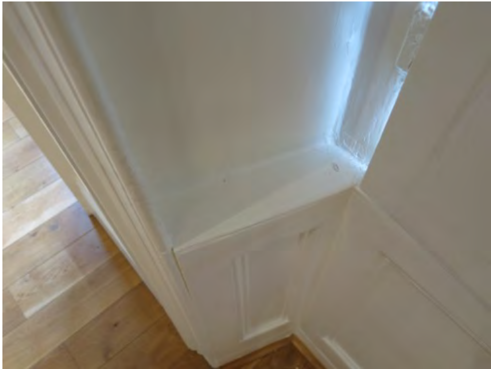
Figure 15: View with the shutters open looking at the shutter box, window architrave and panelling below
