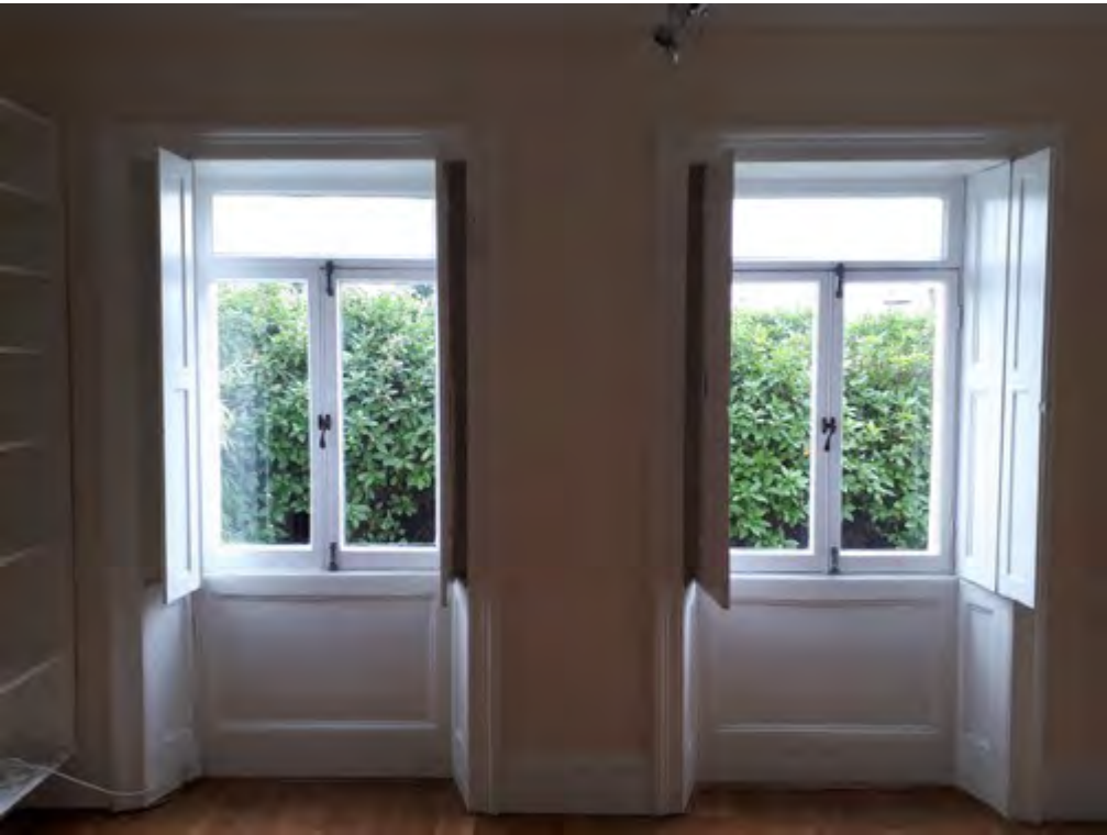
Figure 12: Internal view of the ground floor sitting room windows with the shutters open and unfolded. There are two windows facing out through the external front elevation. Both windows show above will have secondary glazing installed internally.
