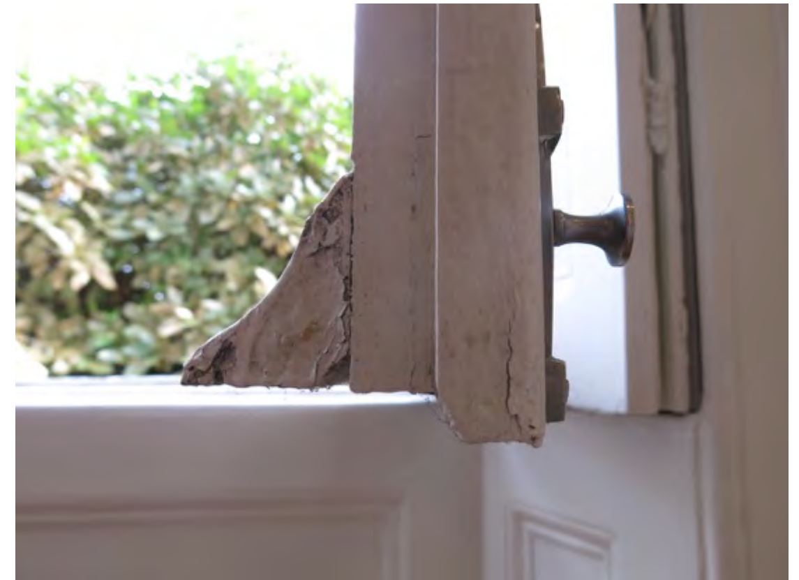
Figure 19: Detail of the window casement and drip moulding. This is an example of a modern (post WWII) replacement which replicates earlier casements
