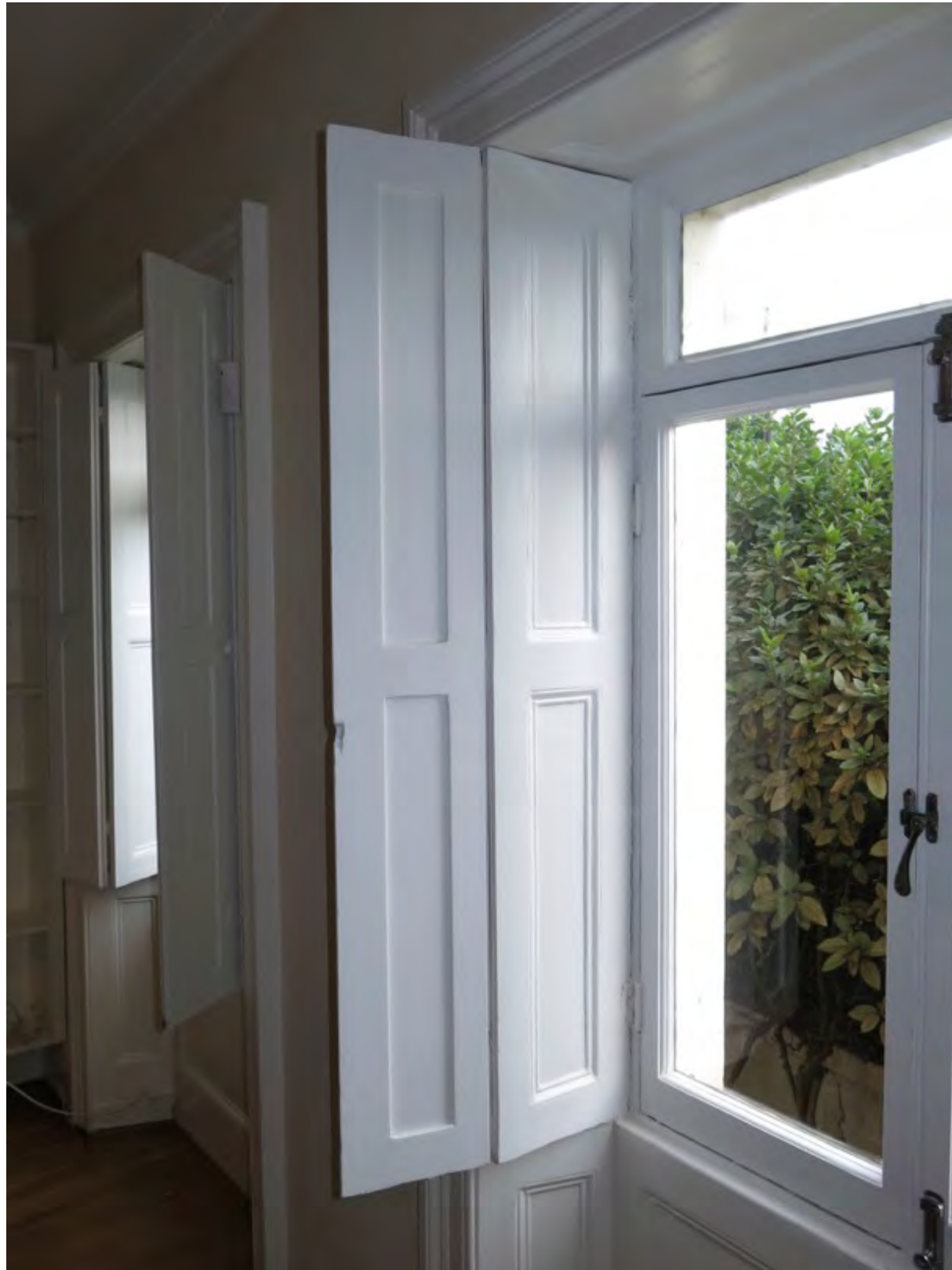
Figure 18: View looking at the unfolded shutters with casement window and fanlight above. The use of casement windows with a fanlight is an unusual format and sash windows are more typical of this period (1824-32). Some of the casements are relatively modern replacements with sharper mouldings and fewer paint layers and float glass.
