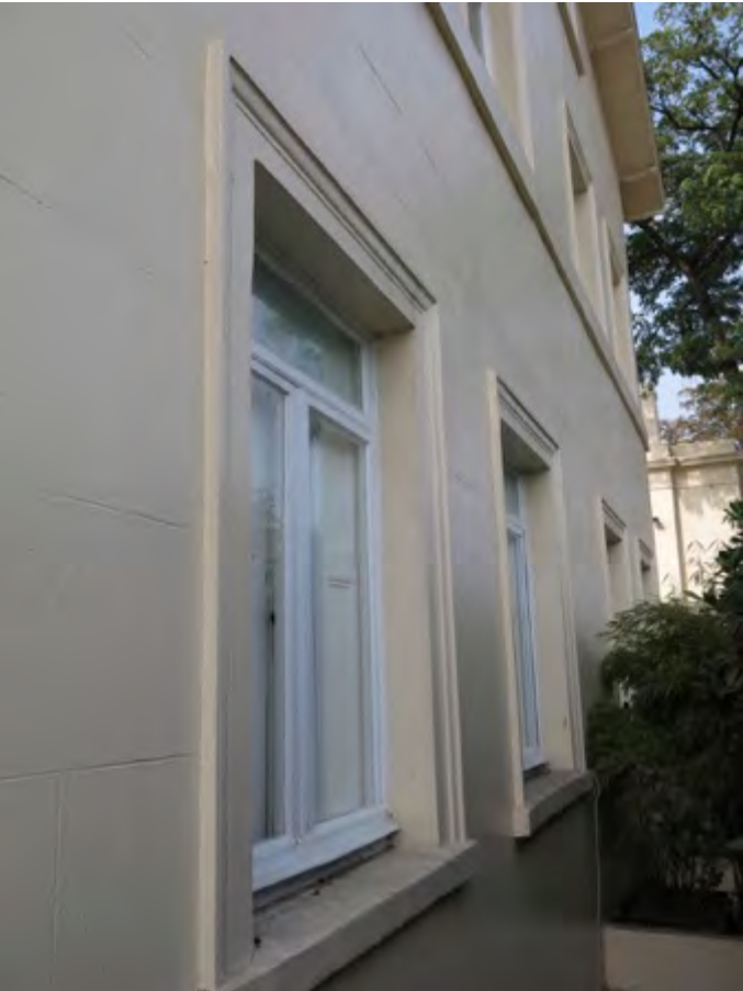
Figure 21: External window elevation with stucco window architrave and ashlar lined wall stucco
