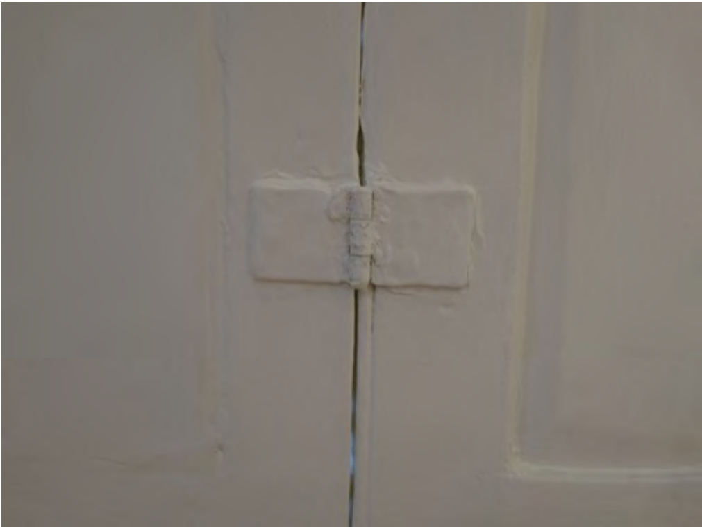
Figure 17: An original shutter hinge covered by numerous paint layers. Some of the fixing screws have been replaced with modern counter sunk cross head screws
