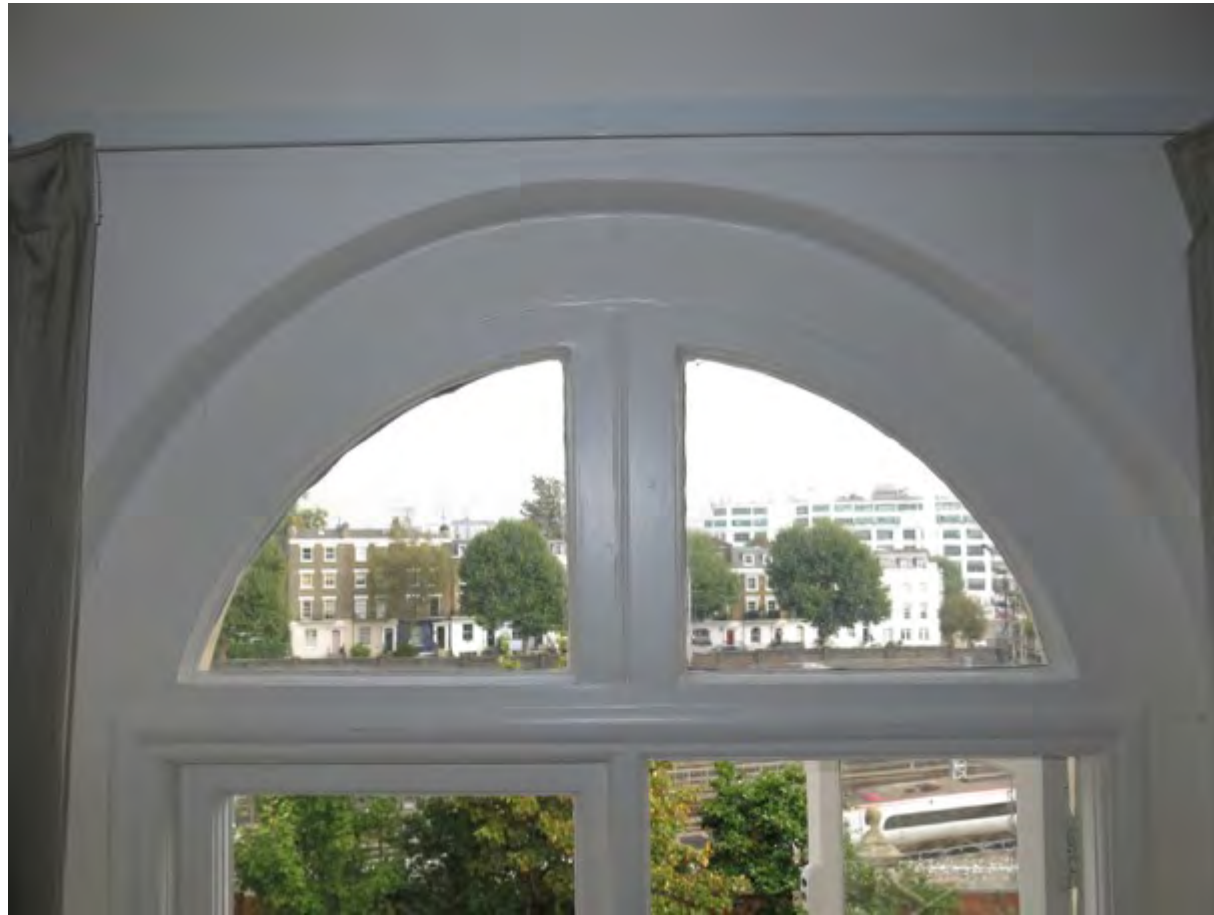
Figure 28: Detail of the fanlight. The presence of a segmental arched window at first floor levels adds weight to the discussion that Nash's original design was based on casement windows. This window format and size is very difficult to achieve with a sash window and would result in a very small opening sash which is visually unsatisfactory.
