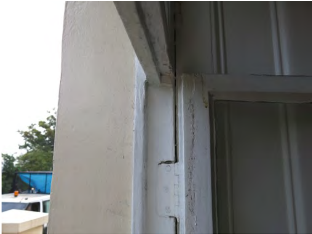
Figure 20: Detail of the window frame and fanlight transom. Note the cast iron butt hinges on the casement
