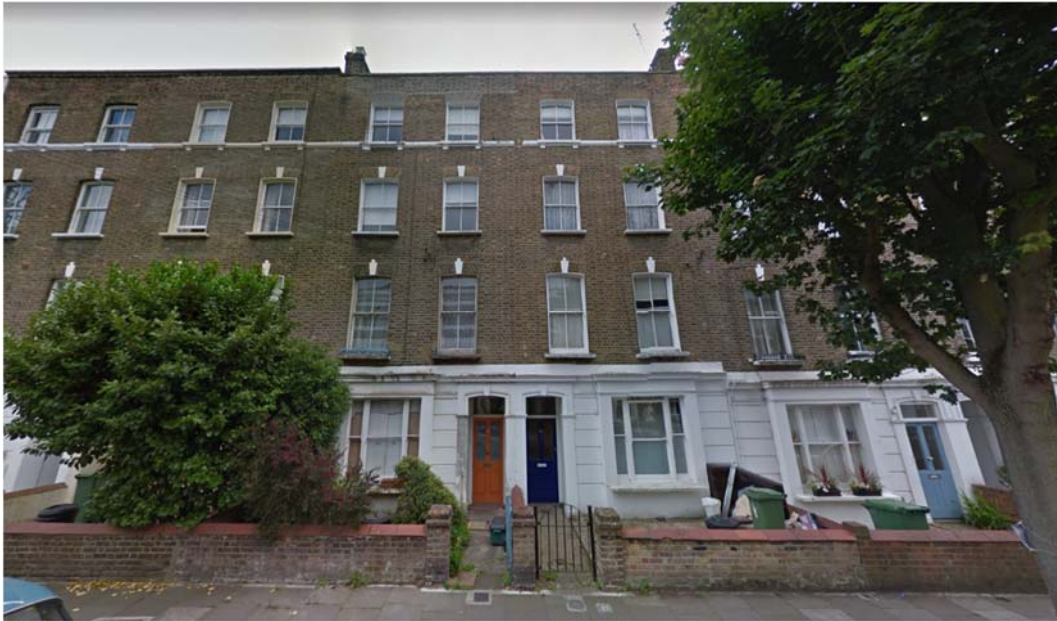
Figure 1: 52 and 54 Falkland Road as existing from the street.
