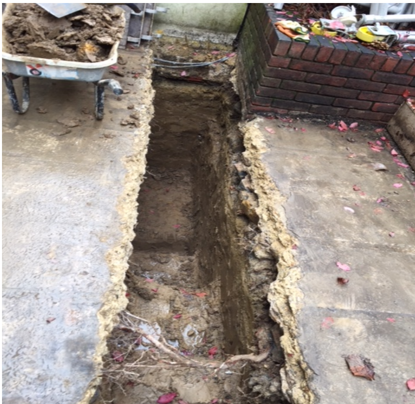
PHOTO 2: the single root of less than 25mm diameter in the trial trench
