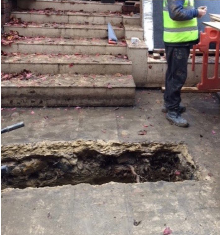
PHOTO 1: position of trial trench and single root
