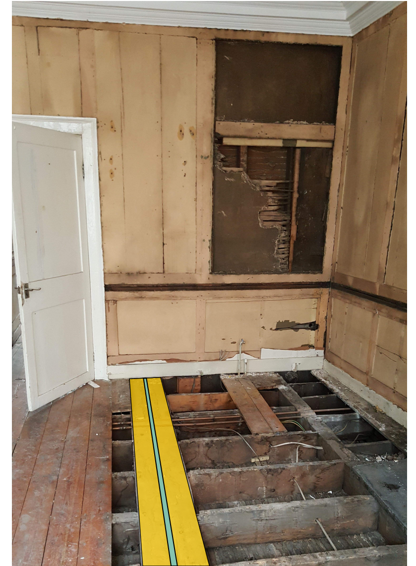
Figure 4, Front Floor Beam To Be Strengthened (Indicative)
