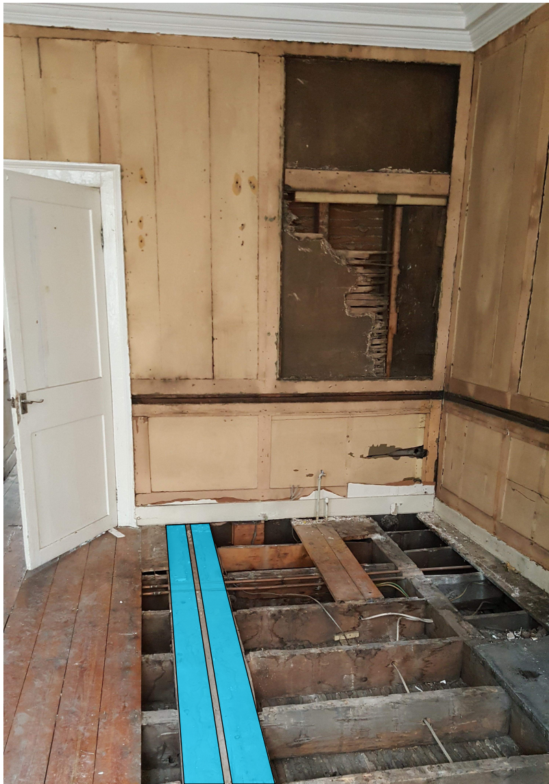
Figure 5, Front Floor Beam To Be Strengthened
