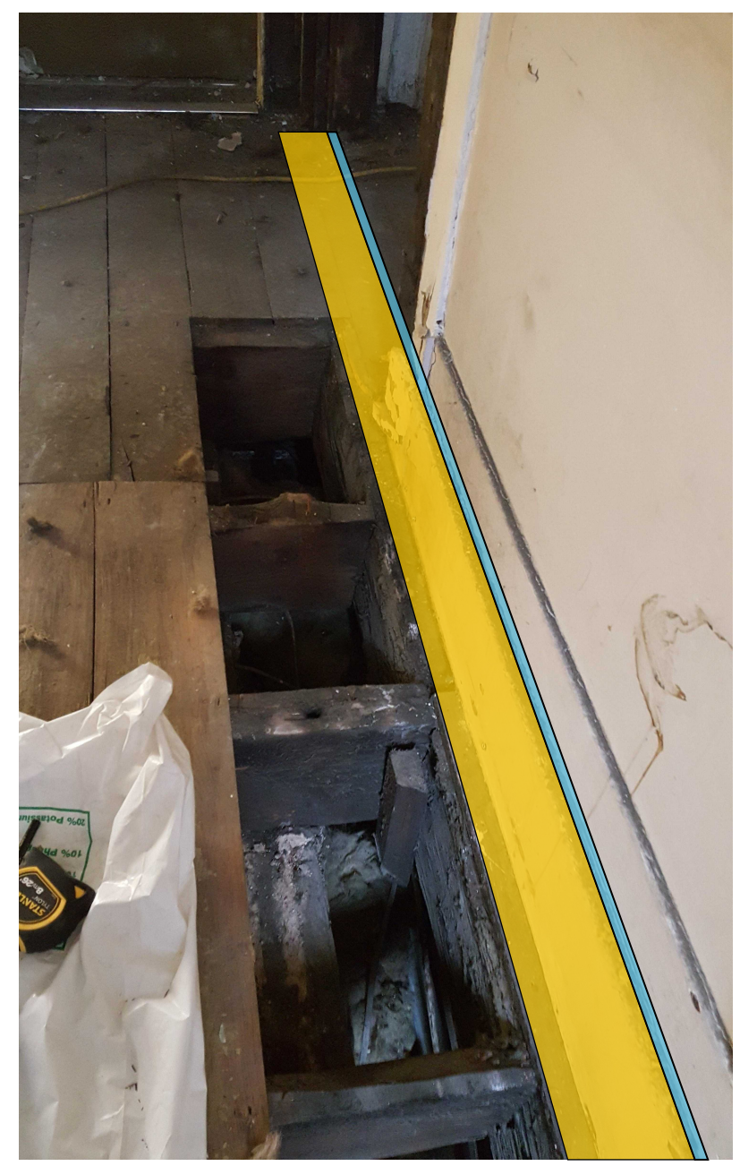
Figure 5, Rear Floor Beam To Be Strengthened (Indicative) Note: Strengthening to opposite side of wall shown
