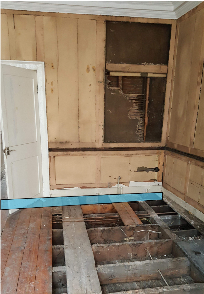
Figure 1, Spine Wall Strengthening Location (Indicative)
