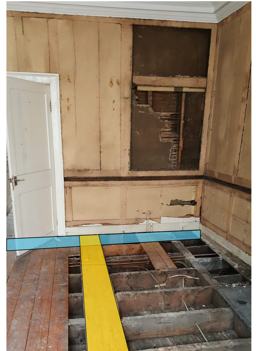
Figure 3, Floor Beam To Be Re-supported (Indicative)
