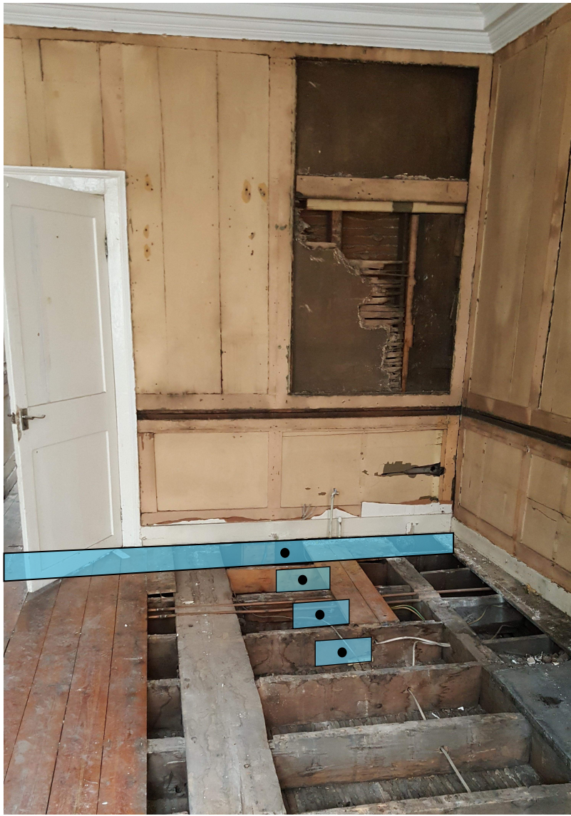
Figure 2, Spine Wall Strengthening Location (Indicative)
