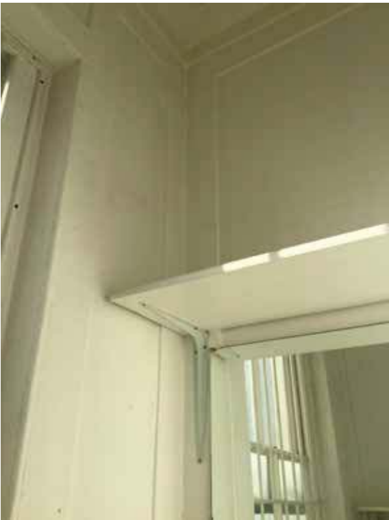
Existing First Floor Closet Wing Cornice and panelling remains much intact, however, shelves and partition detract from the wing
