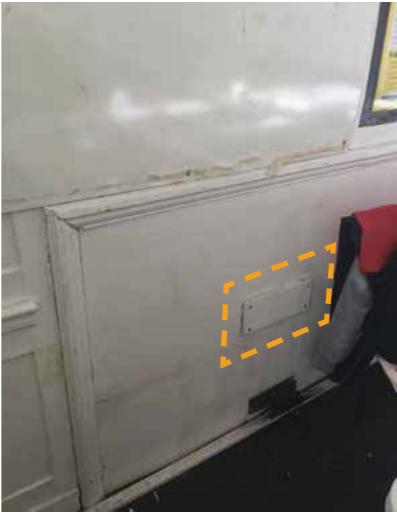
Example of previous services' cut-outs in existing panelling in no. 7 Denmark Street. This can be reused to allow flush-mounted switch plates
