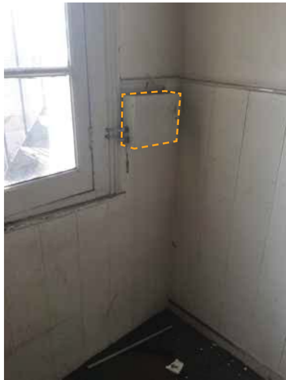
Second Floor half-landing, September 2017, wall-mounted containment with distribution penetrating window frame
