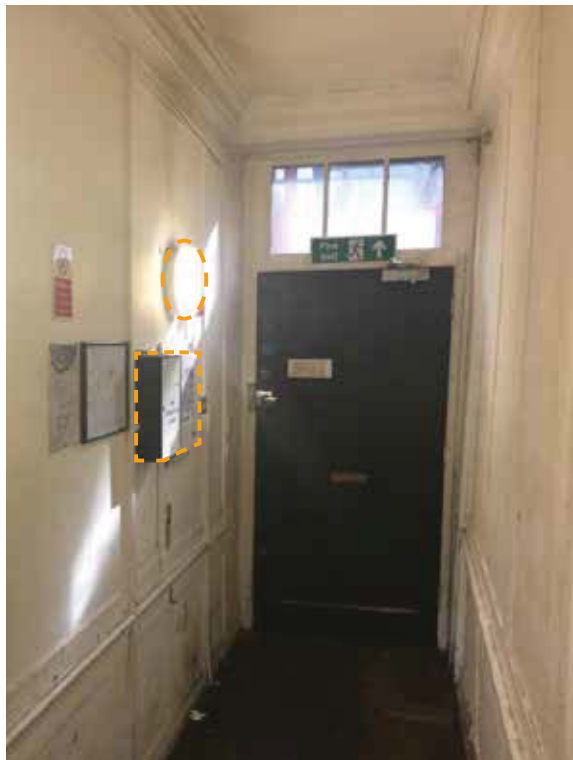
Entrance Hall of No.7, September 2017, following possession showing surface mounted containment and wall-mounted lighting
