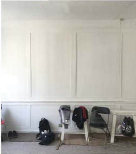
02 X_502 Existing Condition Second Floor Original panelling and dado mostly intact - to be repaired
