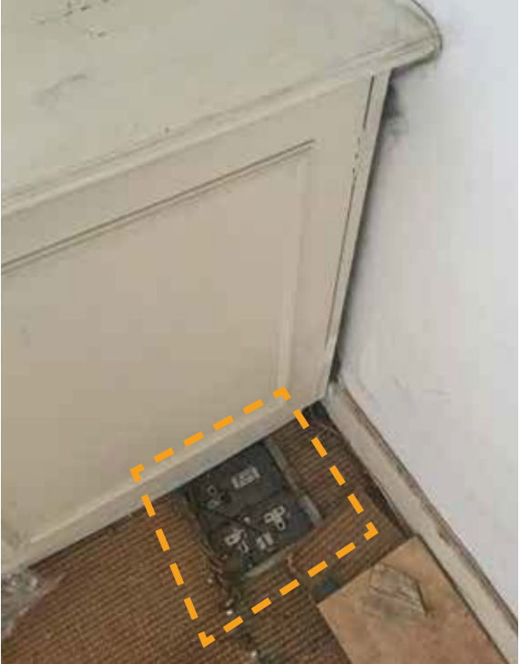
Example of electrical sockets integrated into the floor, to be removed and replaced with flush or surface-mounted switch plates as adjacent.
