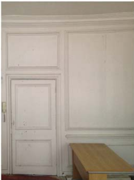
02 X_502 Existing Condition Second Floor Original panelling and dado mostly intact - to be repaired
