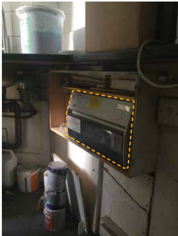
First Floor kitchenette, September 2017, with surface mounted containment
