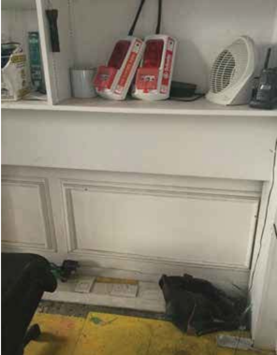
Example of fully intact panelling - surface-mounted back-box and switch plate will be required here
