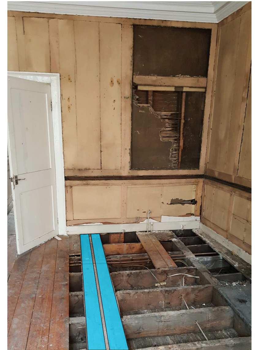
Figure 5, Front Floor Beam To Be Strengthened
