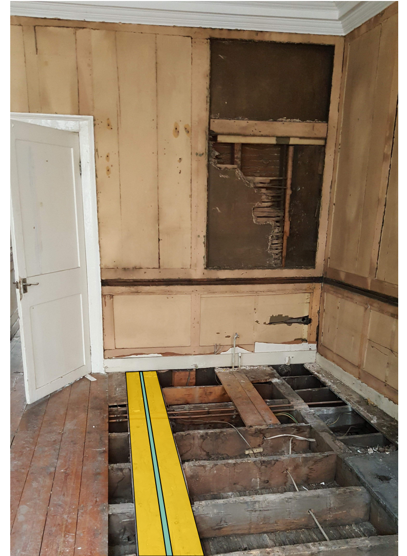
Figure 4, Front Floor Beam To Be Strengthened (Indicative)
