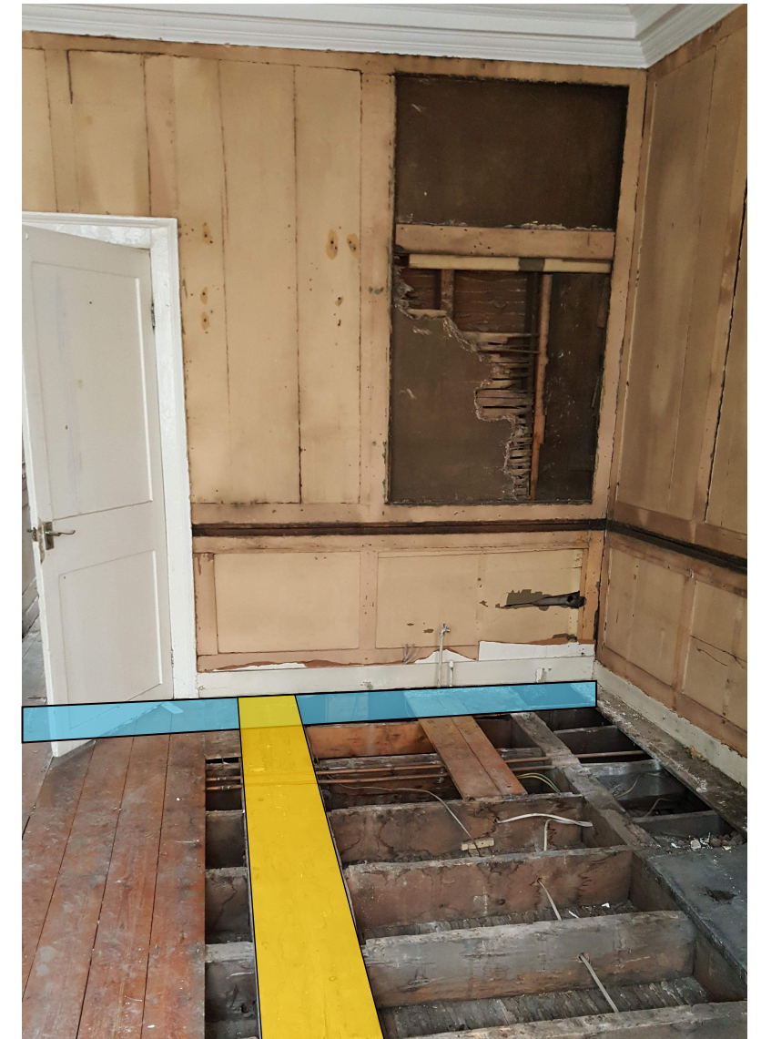
Figure 3, Floor Beam To Be Re-supported (Indicative)
