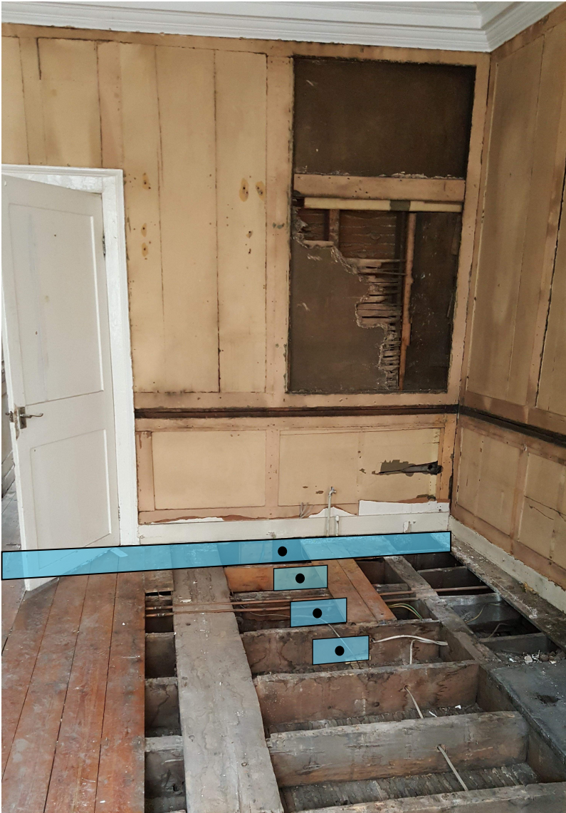
Figure 2, Spine Wall Strengthening Location (Indicative)
