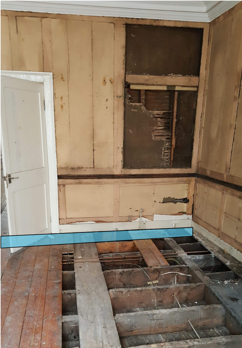
Figure 1, Spine Wall Strengthening Location (Indicative)
