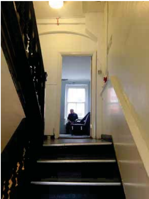
Landing showing signs of floor deflection
