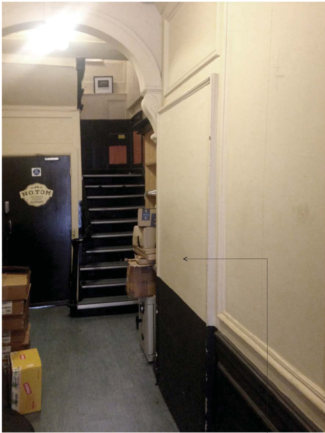
01 X_507 Existing Internal View Ground Floor Hallway - Showing closed-up connecting door and recently revealed panelling
