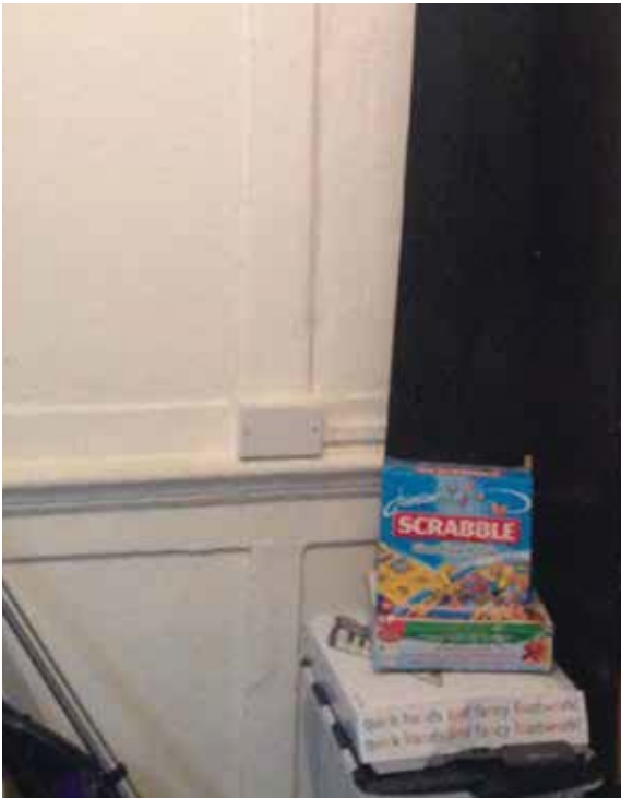
Example of dado level services' cut-outs in existing panelling in no. 6 Denmark Street. Repairs will be required here while switch plates will be located somewhere less conspicuous
