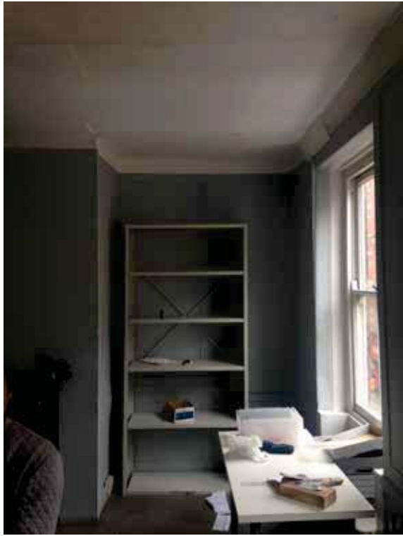
Examples of missing cornice line
