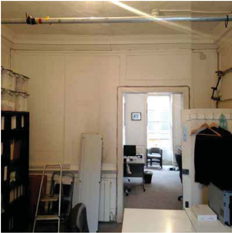
First Floor back room - existing spine wall, large opening to front room a later modification that shall accommodate a new door and be modified to more appropriately suit the panelling
