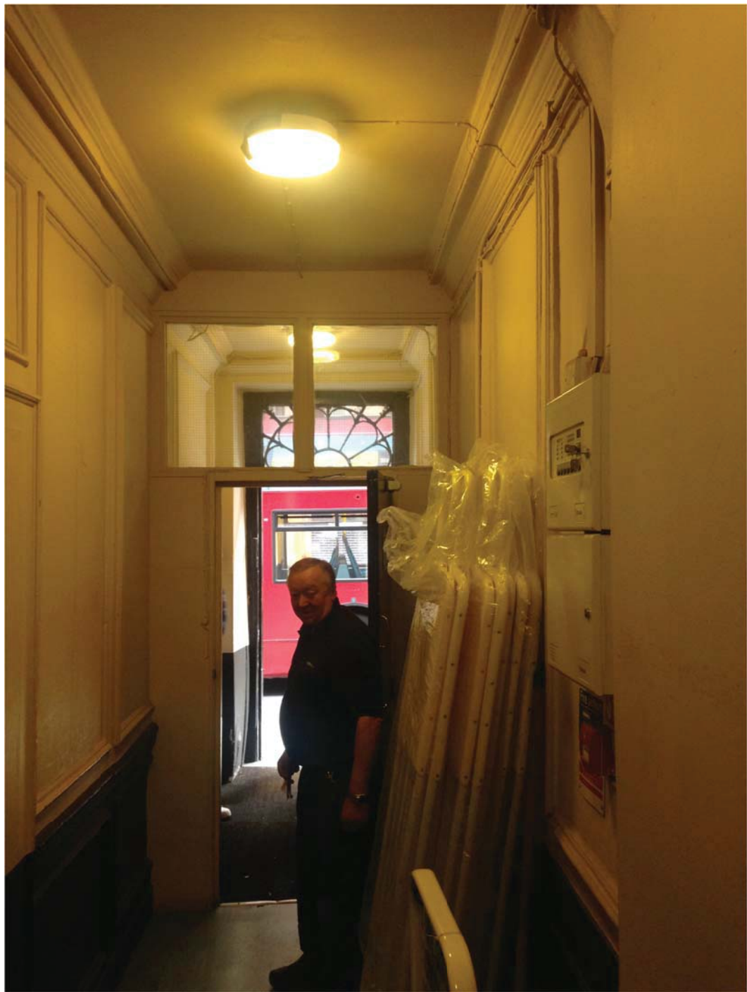
01 X_508 Existing Internal View Ground Floor Hallway - Showing closed-up connecting door and recently revealed panelling
