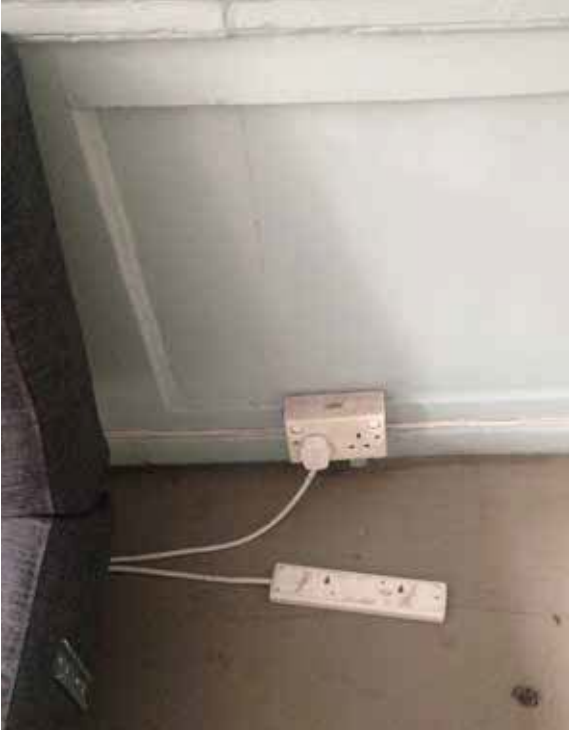
Example of low electrical sockets to be removed to allow repairs to skirting and panelling
