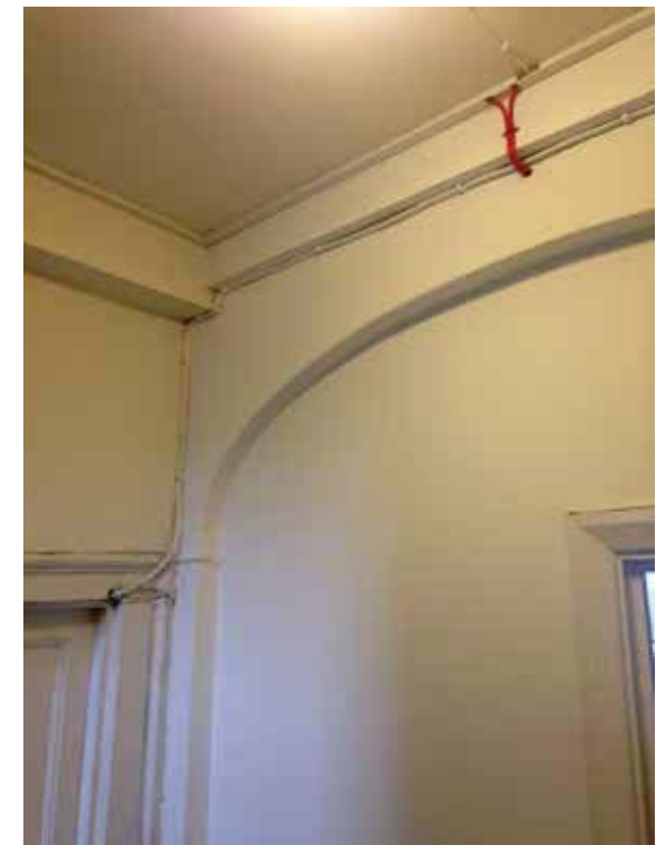
Wiring running across openings and through walls affects the existing fabric. Subsequent modifications to the spaces make for a clash of bulkheads, details and features not in keeping with the period and heritage of the building
