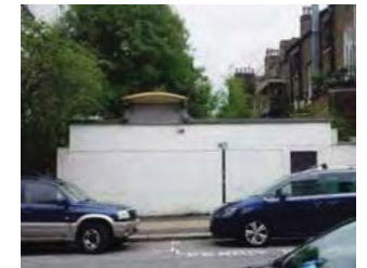
R: Rear of 5 Pond Street
