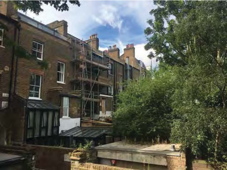
1: View from the existing roof terrace towards south-west
