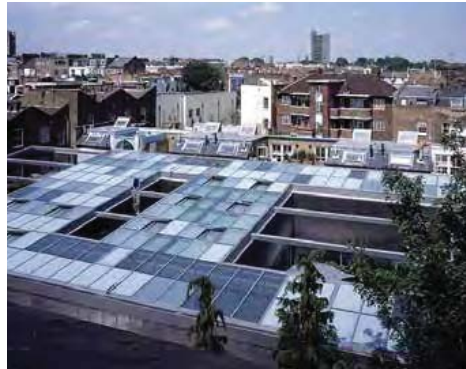
The glazed roof of the house, with openings for open air courtyards
