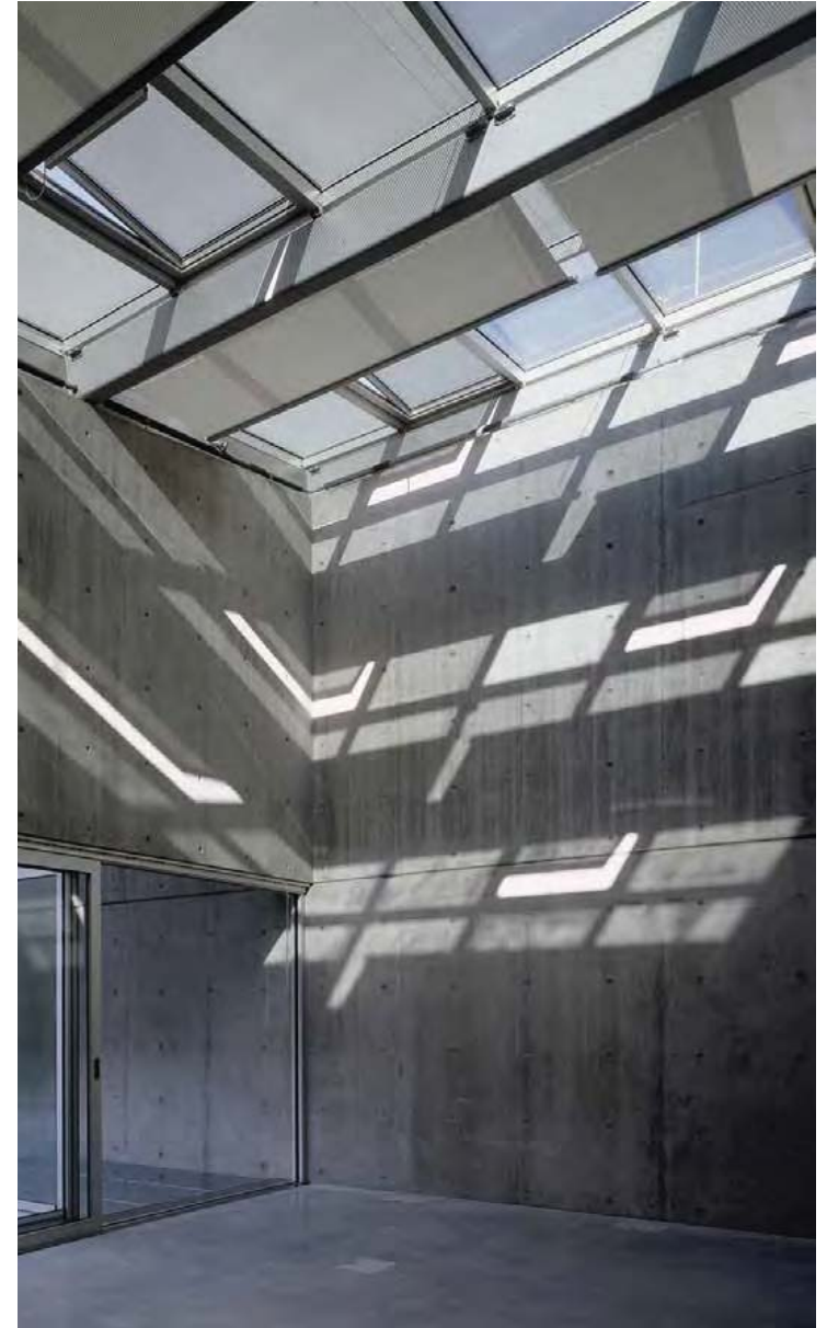
Patterned sunlight on concrete creates a stunning effect in the light house. Electronically operated ceiling blinds offer additional shading to the fritted elements in the glazed roof.
