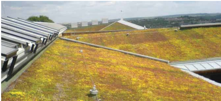
Example of a green roof with sedum
