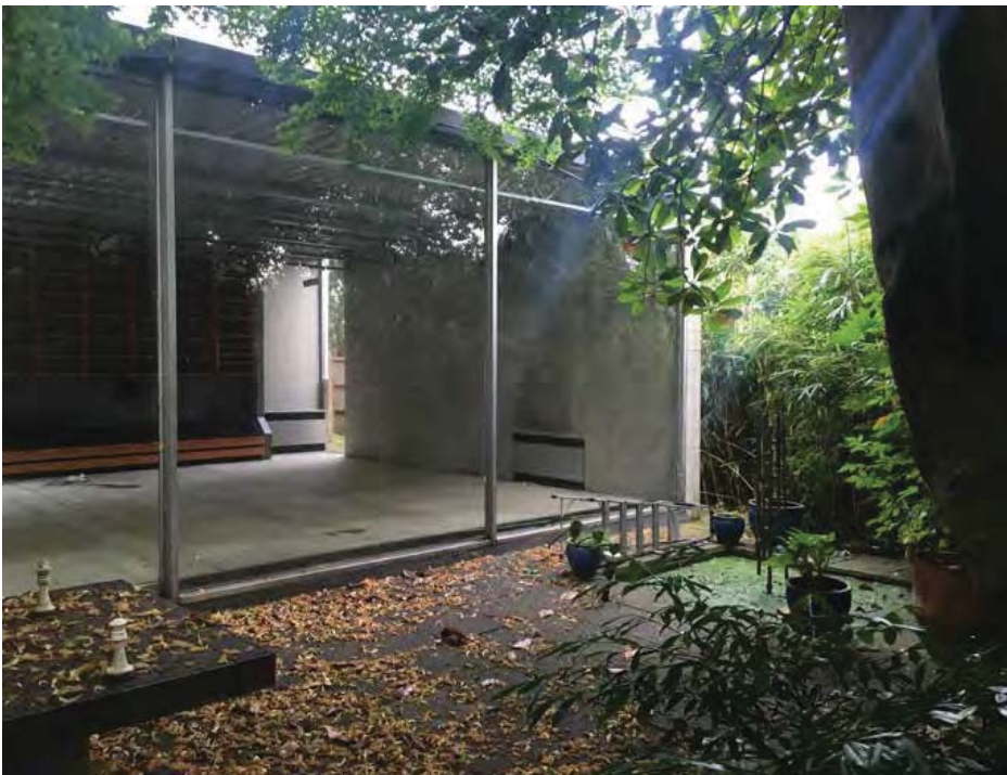
Large sliding glass panels of the extension on east side
