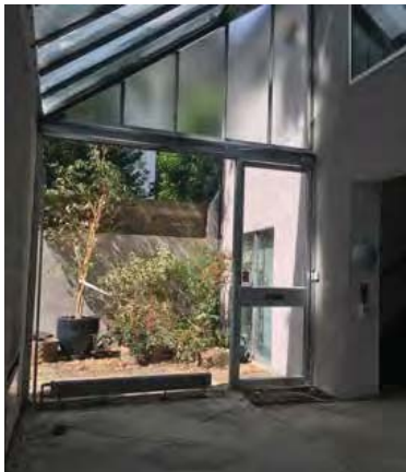
Internal view of the kitchen towards the entrance
