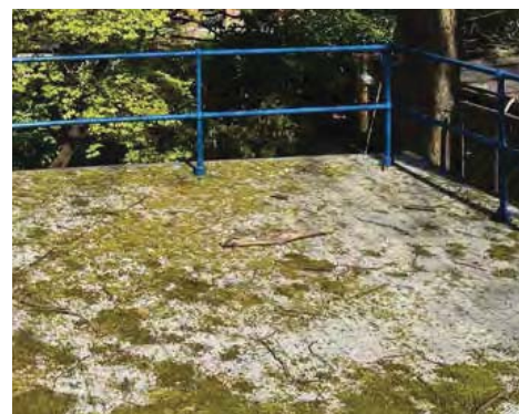
8: Roof terrace with plastic tiles
