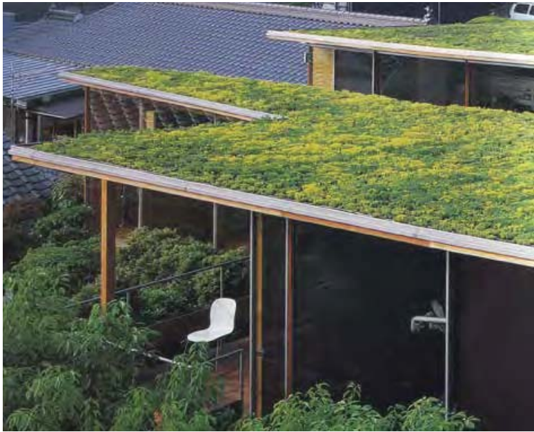
Example of a green roof with sedum
