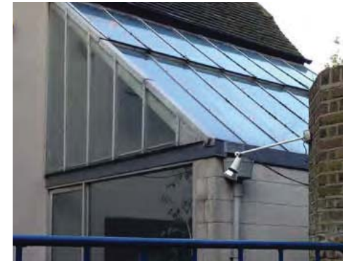
3: Glass door and patent glazed roof
