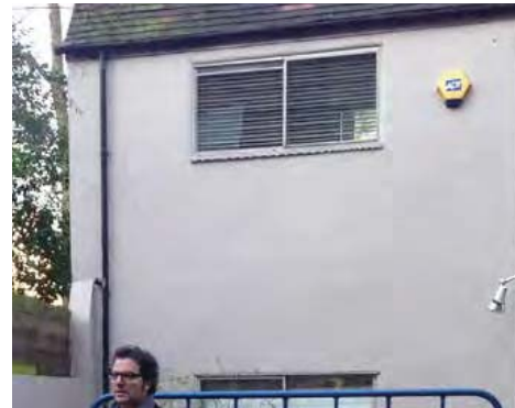
2: Rendered and painted walls with aluminum framed windows
