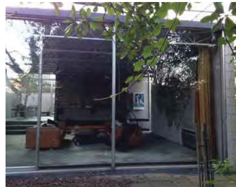
5: Steel framed glass sliding door
