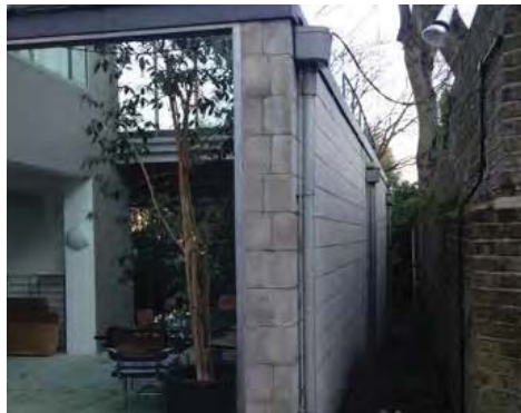
4: Exposed concrete block wall
