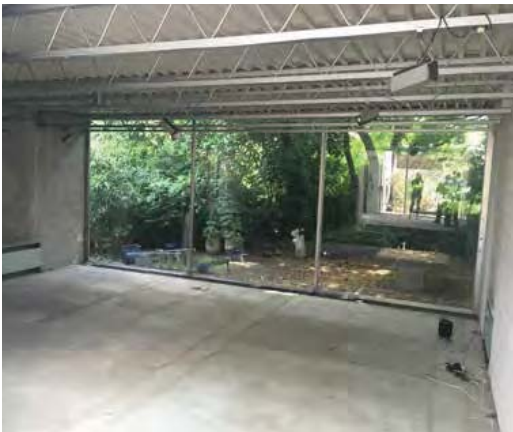
Internal view of the extension towards the garden
