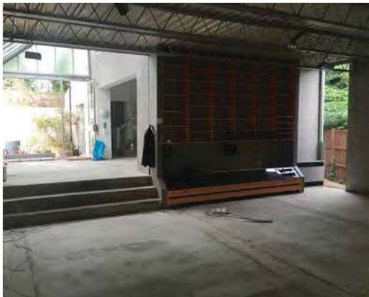
Internal view of the extension towards kitchen
