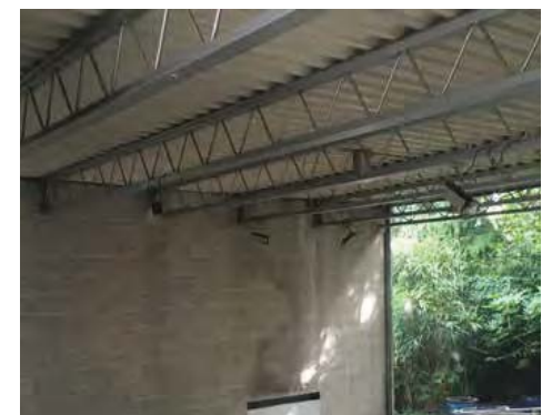
9: Ceiling of living room with steel structure and corrugated aluminium
