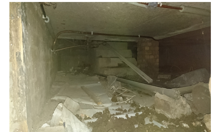
Void from utility room. Beam and block floor with internal masonry pier
