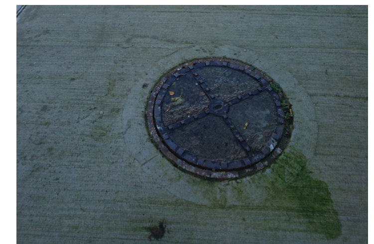
Manhole to rear of 24 Lawn Road
