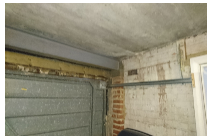
Photo of existing first floor soffit and supporting steel
