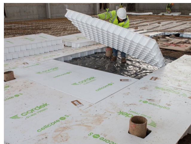
Underslab Heave Protection
