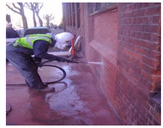
Cleaner undertaking Jos Torc cleaning on brickwork
