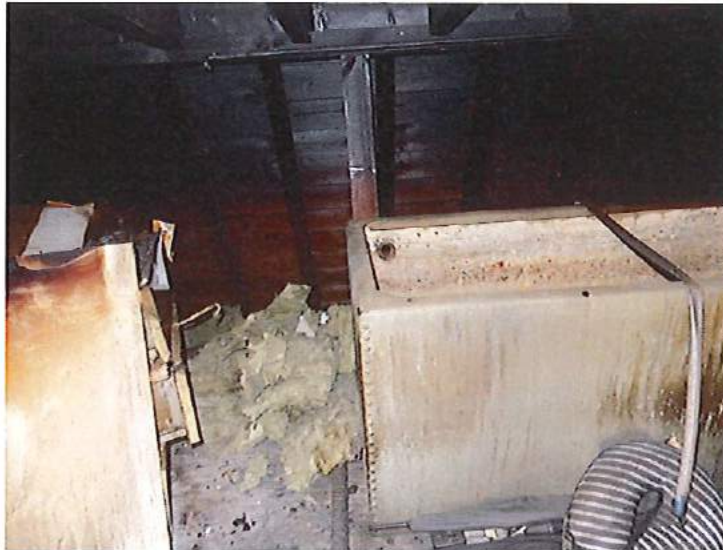
Stored goods in roof space
