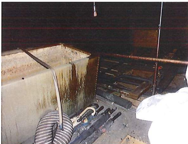
Water tank (assumed redundant?) in roof space
