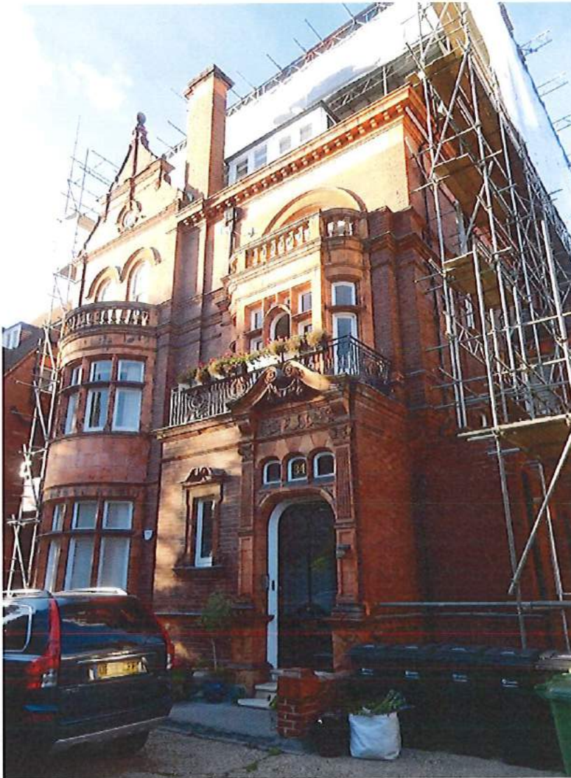
Front elevation showing moulded terracotta pediment / cresting details and unglazed tiles / blocks
