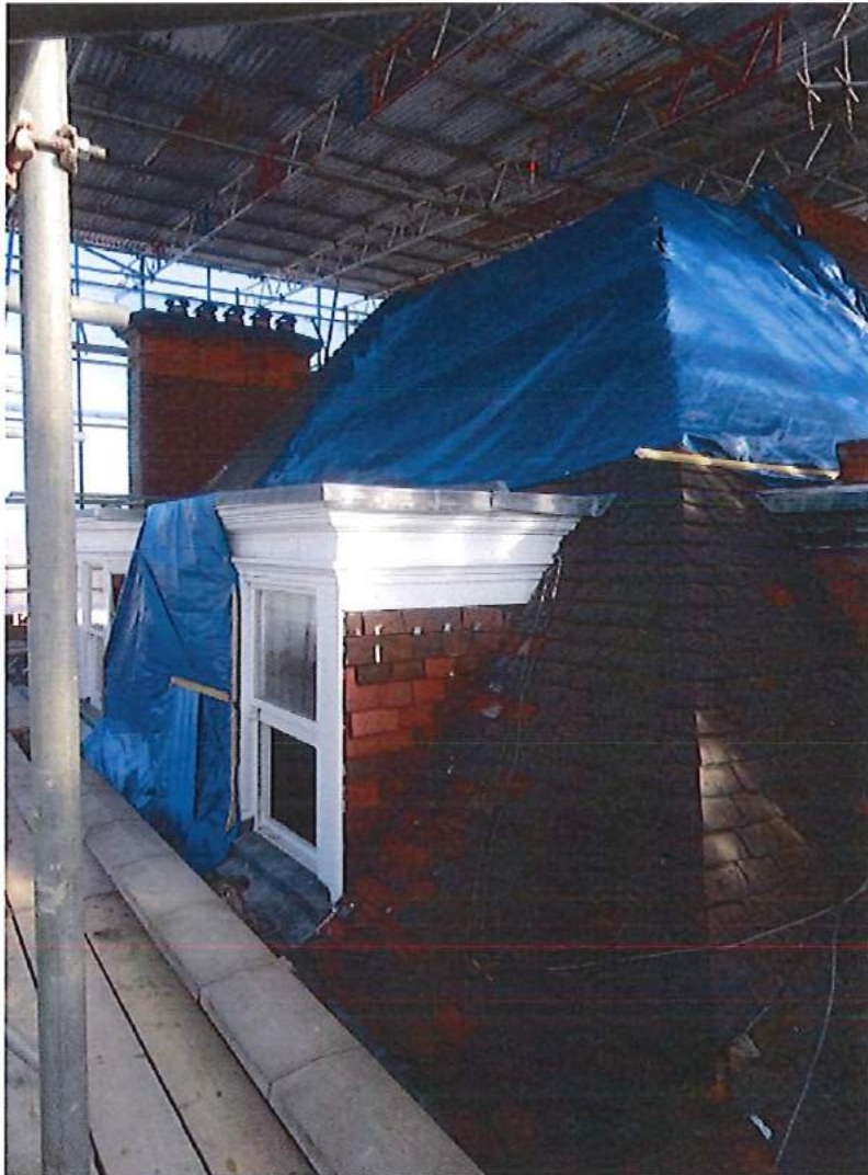
Flat roof to pyramid shaped roof structure
